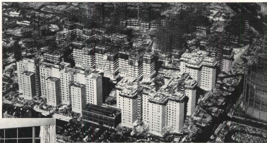
Stuyvesant Town Apartments, New York City, a Development of the Metropolitan Life Insurance Company
