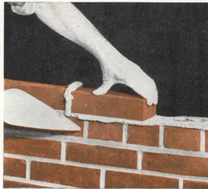
The brick should then be pushed into place.
