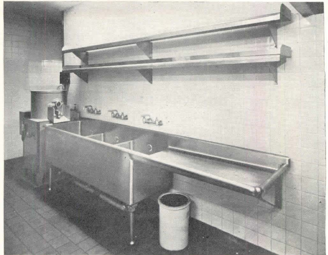
Note soaking sink and pre-flush for swill. Right: Mayflower preparation equipment; note vegetable parer at far end of sinks
