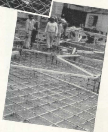
Reinforcing rods for floor slab. Piles can be seen below.
