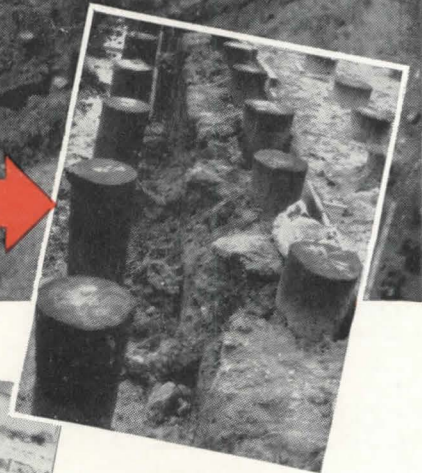
Piles in trench will be capped by wall; others by floor slab.
