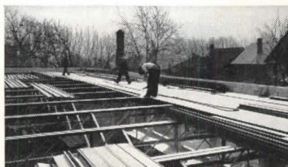
Application of "Ferrobord" Steeldeck
