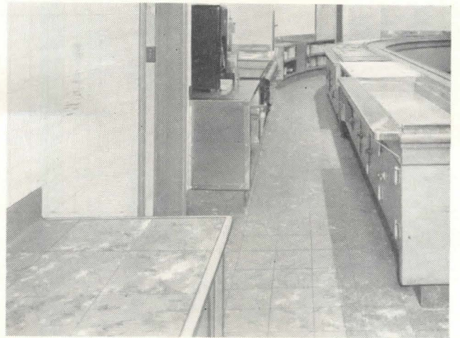
Asphalt tile , although limited in its practical application to surfaces where numerous joints are not objectionable, has advantages in its thermoplastic qualities. It can be heated and bent to form a dirt-free cove at the junction of vertical and horizontal surfaces.
