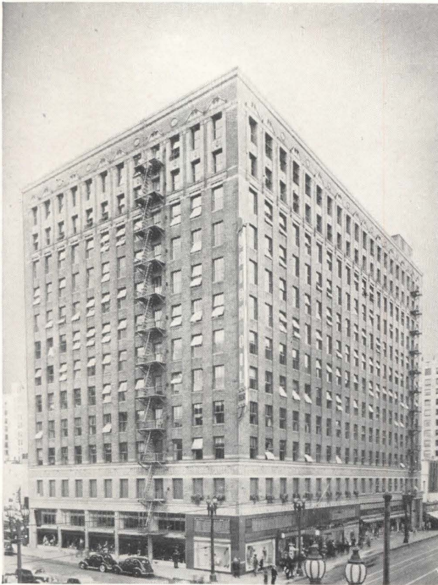
Union Oil Building, Los Angeles, erected in 1923 and originally equipped with six car-switch elevators.
