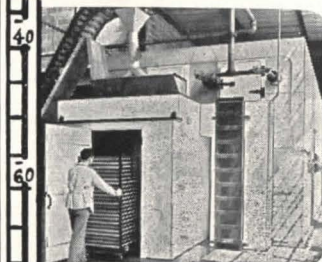
Frick-Freezer Tunnel operated at -35° F. at Lancaster, Pennsylvania.
