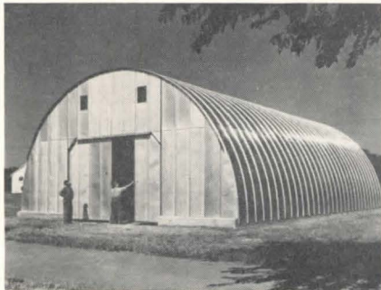
Aluminum framing and sheathing are used in prefabricated arch-roofed structure
