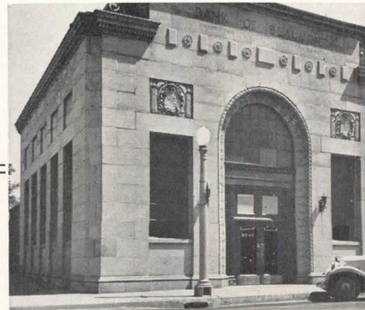
"Very satisfactory in all respects," agrees W. D. Vice President and Cashier of the Bank of Bea California, which is kept cool in summer, comfortable and warm when needed, by the Servel unit.
