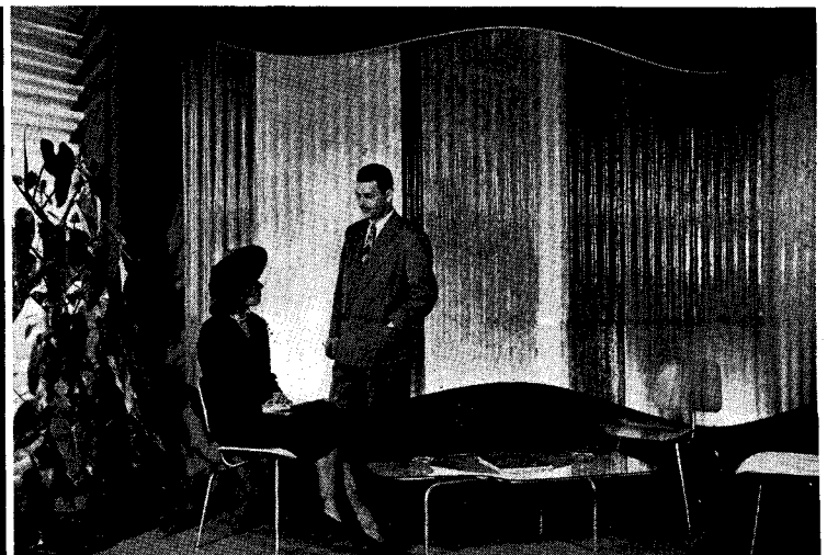
Glass-and-plastic laminated panels are flexible and can be bent to fit curved surfaces; come in colors, translucent or opaque
