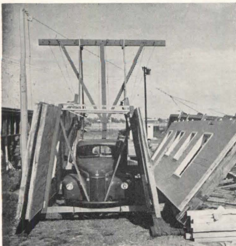
Fast assembly of Florida homes: walls are loaded four at a time on specially rigged truck (left), taken to site and unloaded directly from truck to foundation (below)
