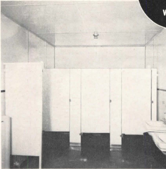
Sparkling, sanitary washrooms are important! Easy-to-clean Marlite is the answer.
