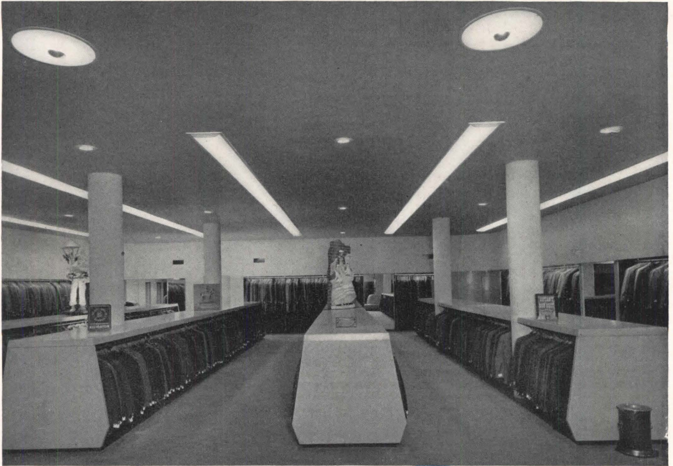
Men's Clothing Dept., Greenfield's Store, St. Louis, Mo. Five continuous rows of nine fixtures each are recessed in the 11'2" ceiling to produce approximately 40 foot candles maintained. L-I-N-O-L-I-T-E Series 17 two lamp troffers with curved Holophane Controls (17-248) were used for this installation. Architect: Meyer Loomstein.
