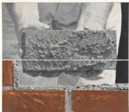
Then the mortar will stick to the brick on top of it as well as to the brick below it.
