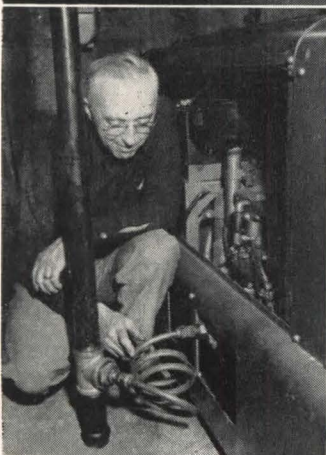
Edgar Shaeffer, Manager, Roxy Theatre, with Onan Standby System. Plant runs on natural gas.
