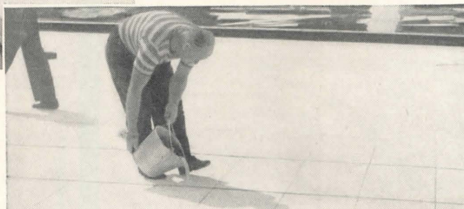
EASY TO FIT. Kaylo Insulating Roof Tile can be cut and fitted with ordinary hand or power tools. Picture above shows example of entrant cut made to fit around stack.
