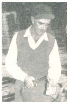
The workman is holding a slab of pumice concrete in his bare hand while heating the face of the slab to fusion with a gas torch.
