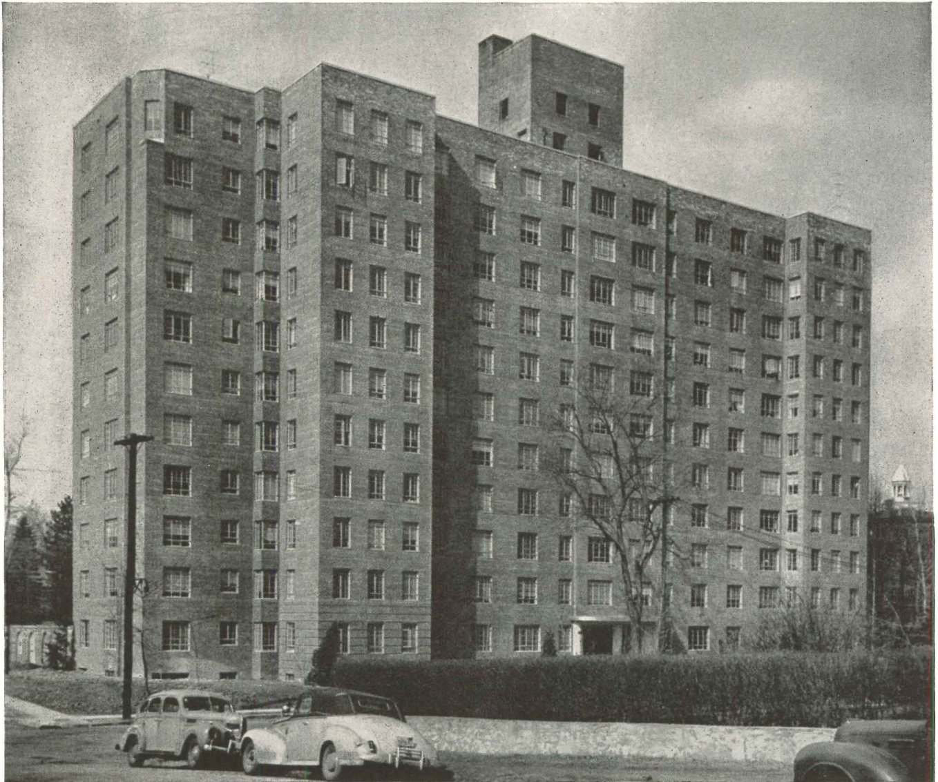
Architect: Rosario Candela, New York. Engineer: Louis d'Antona, New York. Steel Fabricator and Erector: Schacht Steel Construction, Inc., New York.
