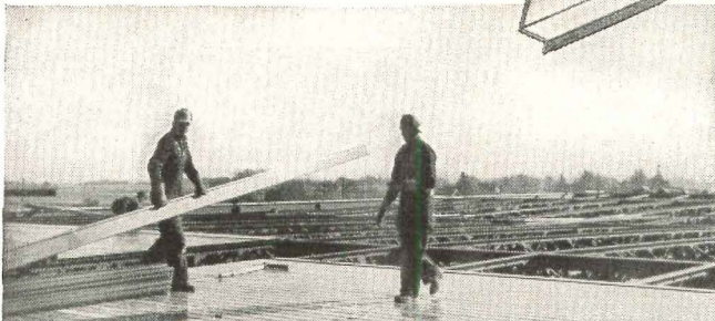
Truscon Ferrobord Steeldeck being installed in the new Automatic plant, Maytag Washing Machine Company, Newton, Iowa. Arthur H. Neumann & Bros., Inc., Des Moines, Architects, Engineers, Contractors.
