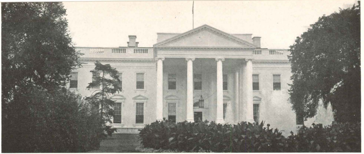
The White House as it looks today from Pennsylvania Avenue; present rebuilding program will preserve this facade
