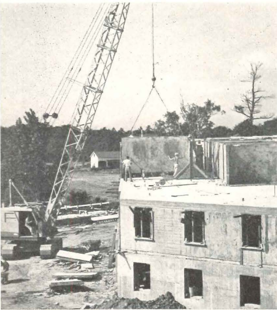
Photo, left: setting up precast wall slabs at the Univ. of Vermont. Simple wood bracing held slabs in place; floors were poured in place in forms built over slabs. Details below photo show typical dormitory construction. Bottom right: some of the first dorms built at the Univ. of Connecticut
