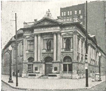
Main Office of Indiana National Bank, Indianapolis. Equipped when originally designed by D. A. Bohlen & Son with Webster Steam Heating System. In 1947, Strong Brothers, heating contractors, modernized the installation by installing Webster Moderator System.
