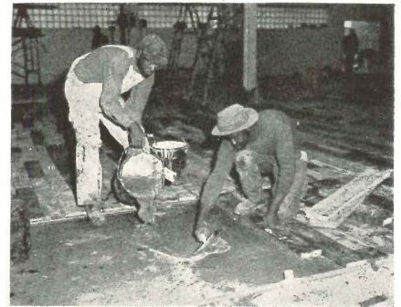
Special adhesive cements subflooring to concrete, eliminates need for sleepers
