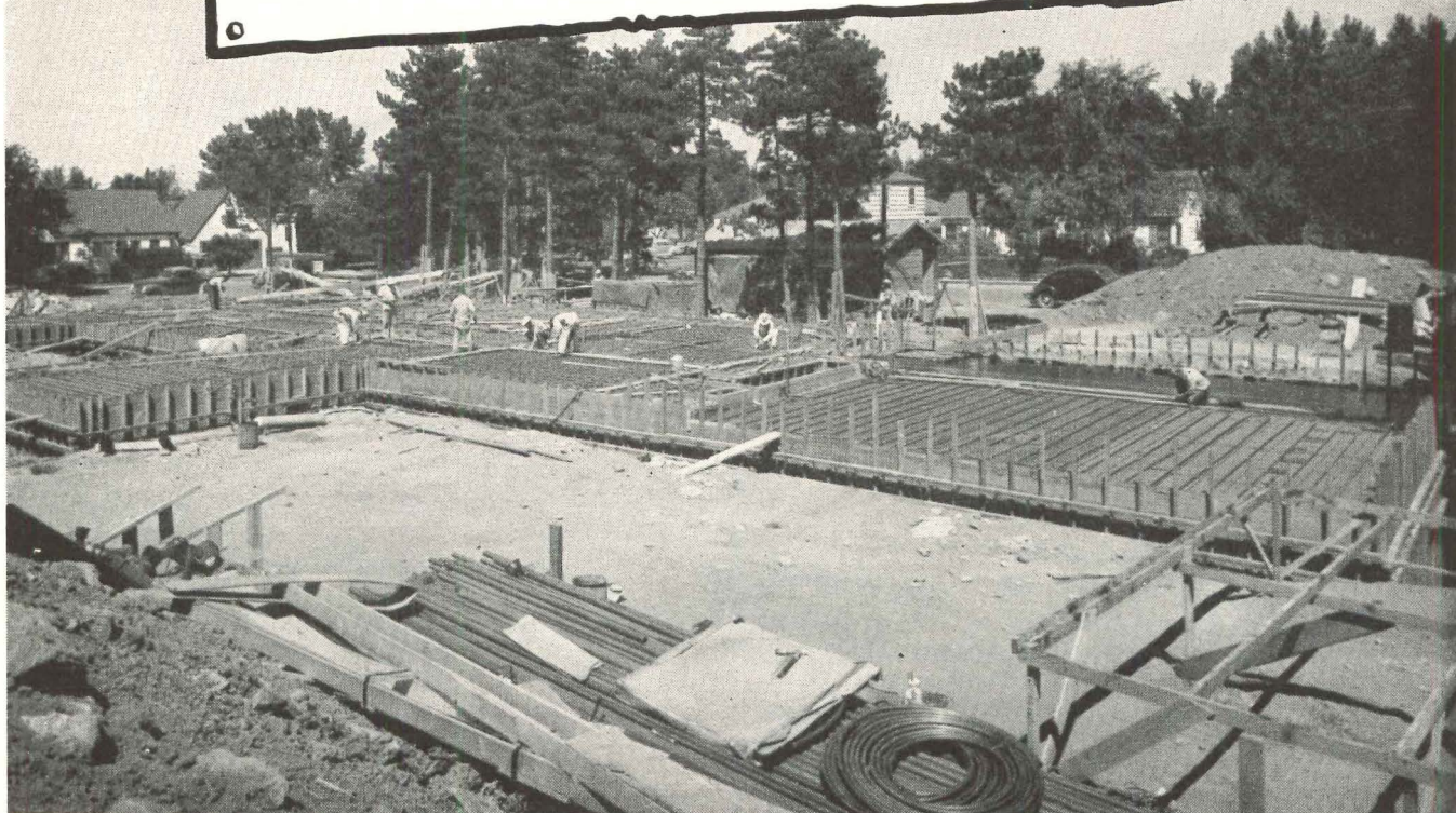
11,000 feet of Revere Copper Water Tube were used in the radiant panel heating system. The building has 9 zones, with each room controlled by individual thermostats. Revere Copper Water Tube was also used for hot and cold water lines, and Revere Sheet Copper for roofing.
