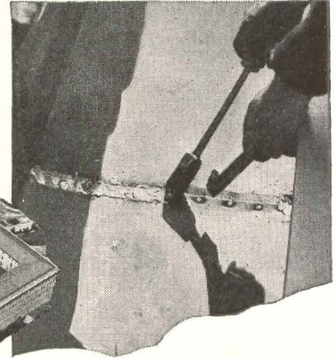
FOR PERMANENT PROTECTION, the old gutters have been replaced with gutters made of strong, corrosion-resistant and economical Monel Roofing Sheet. Here a worker solders a riveted seam in the gutter lining.
