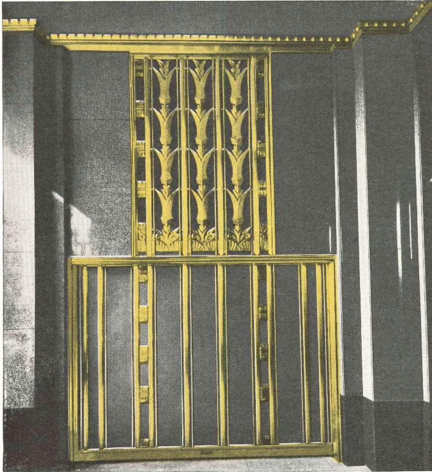
View of vertical sliding door (closed) that conceals cigar stand in lobby of Mirror Building. Anaconda Architectural Bronze Extruded Shapes are employed in sliding door and ceiling moulding (which has been machined). Architect, Rowland H. Crawford, Beverly Hills; General Contractor, P. J. Walker Co.; bronze work by Cochran Izant Co.—both of Los Angeles, Cal.
