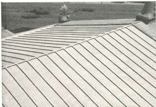
Finished double pitched roof on front.
