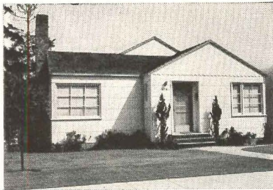
For lapped-siding, some stock sizes other than 4 x 8-foot are ideal. Eighteen inch siding, for example, cuts out of 3-foot wide panels exactly.
