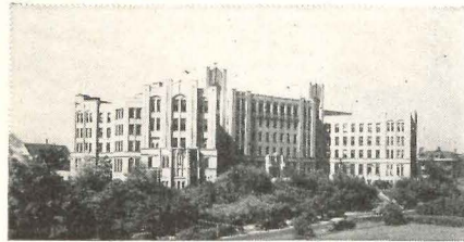
Children's Hospital, Cincinnati—equipped with Worthington Air Conditioning
