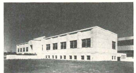
Plant for Turner-Newall (Canada) Ltd., at Montreal covers 10 acres, is devoted to manufacture of asbestos products. Designed by E. C. Miller of T. Pringle & Son Ltd., consulting engineers.
