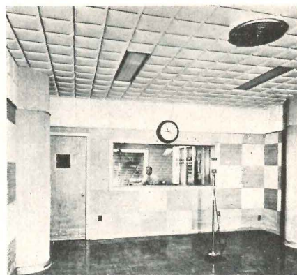
Cotton acoustical tile in radio studio
