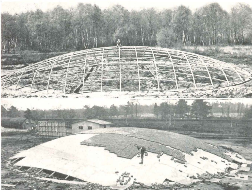
Left, above: rib structure of experimental aluminum roof in position at ground level. After tests for deflection readings were made (directly below) by covering the roof with bricks, dome was stripped for distortion readings (left, below)
