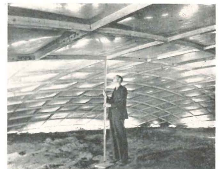
Left, above: rib structure of experimental aluminum roof in position at ground level. After tests for deflection readings were made (directly below) by covering the roof with bricks, dome was stripped for distortion readings (left, below)
