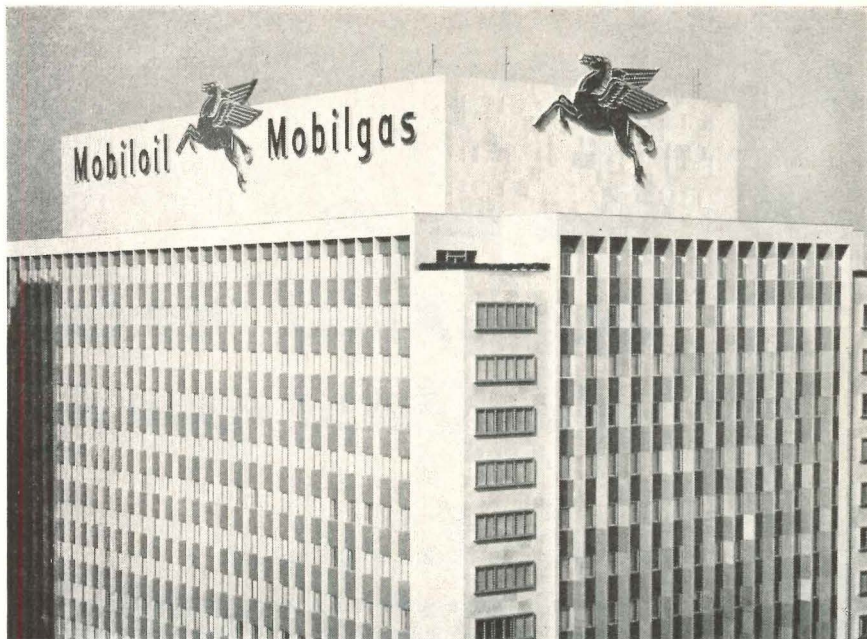
GENERAL PETROLEUM BUILDING, LOS ANGELES, CALIFORNIA
