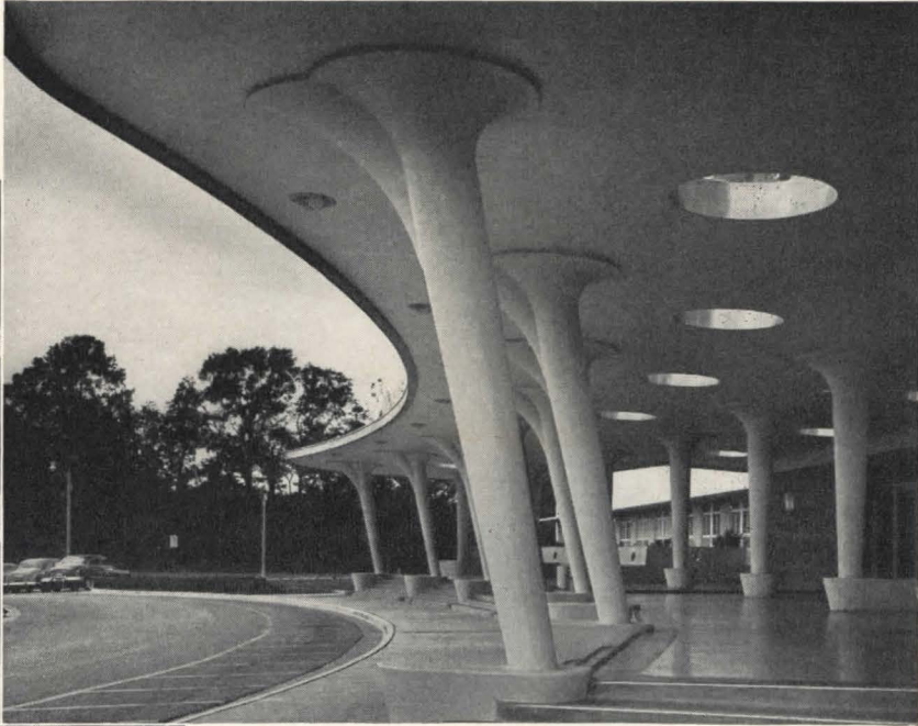
Mobile Infirmary, Mobile, Alabama Platt Roberts & Company, Architects
