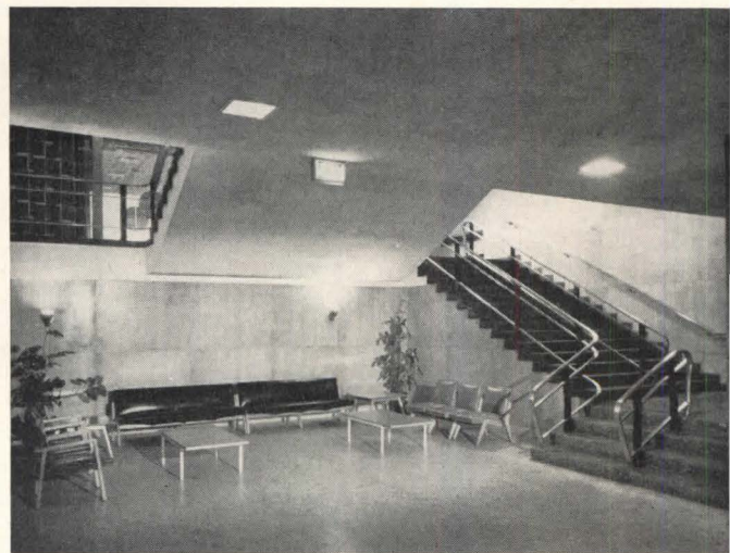
Principal stair has terrazzo treads and risers, satin-finished aluminum handrails, ends at ground floor level in lobby for ballroom
