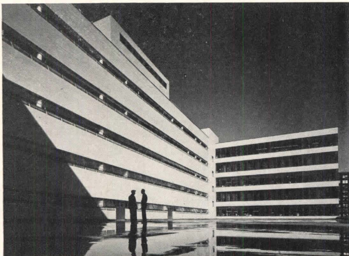
Florsheim Shoe Company General offices and Main Factory, Chicago; Shaw, Metz & Dolio, Architects-Engineers
