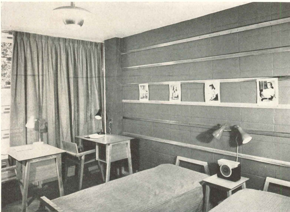
To study and demonstrate the typical dormitory room a full-scale mock-up was built and completely equipped. In plan, rooms are paired with a storage wall (containing wardrobes, dressers, shelving and lavatory) between. Other walls are painted concrete block. Special radiant panels are installed under windows
