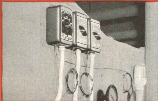
Motor-operated valves (above) and remote bulb thermostats (below)—typical of the over 400 Barber-Colman electric components used for temperature control in Research Tower.
