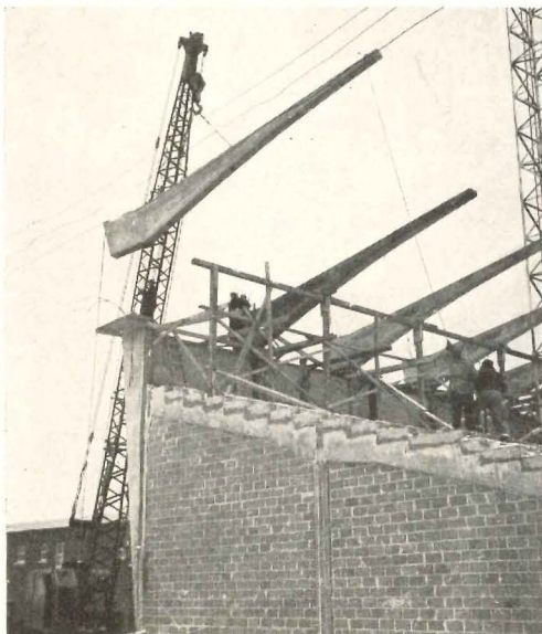
Cantilevered roof beam being lowered into place
