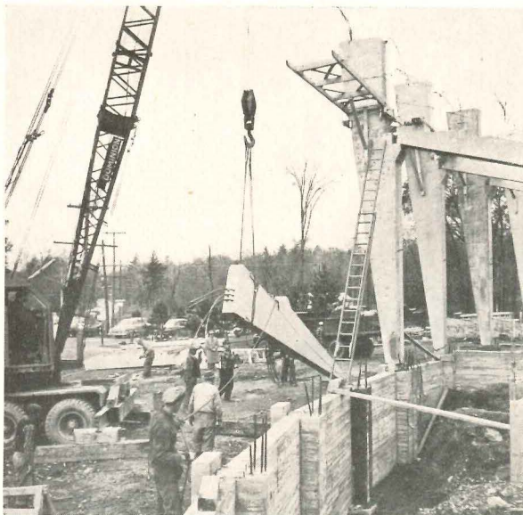
Tapered column, with unstressed cables projecting
