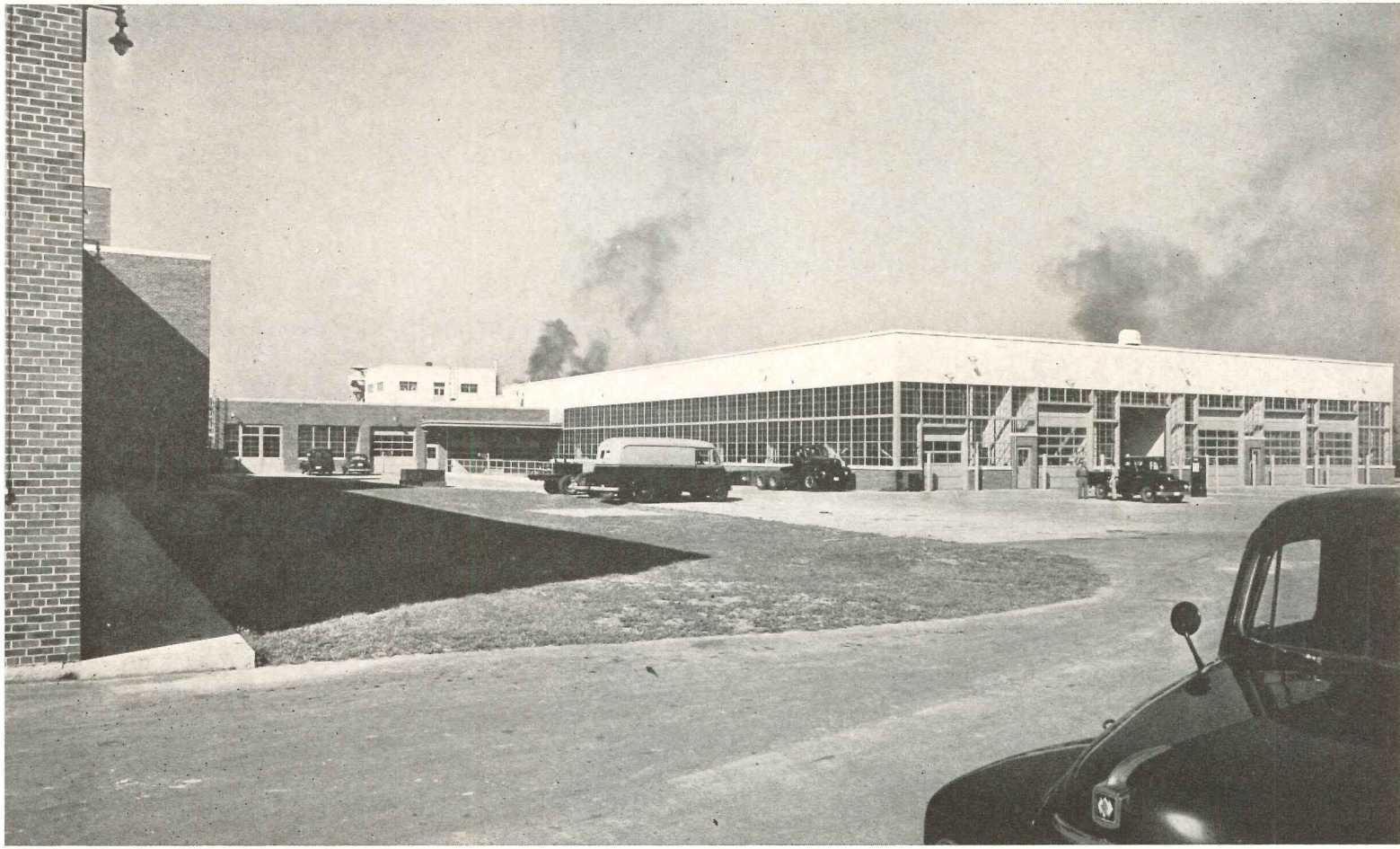
Courts between the wings of the E-shaped building prove useful for access to various sections and parking space for the trucks under study, also for exterior display purposes. Entire building was placed on fill of silty blue clay compacted by sheepsfoot rollers
