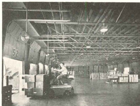
Transcon Lines, Los Angeles, p. 178. Main feature is the suspended wooden roof which has a 35-ft overhang, shielding trucks from hot sun. Two years of planning, including a tour of major terminals, helped simplify and streamline operating procedures
