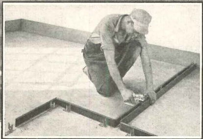
Wheeling Metal Base firmly locks into position on both sides of Floor Clips. Ceiling Runner goes up easily using stub nails or rawl drives.
