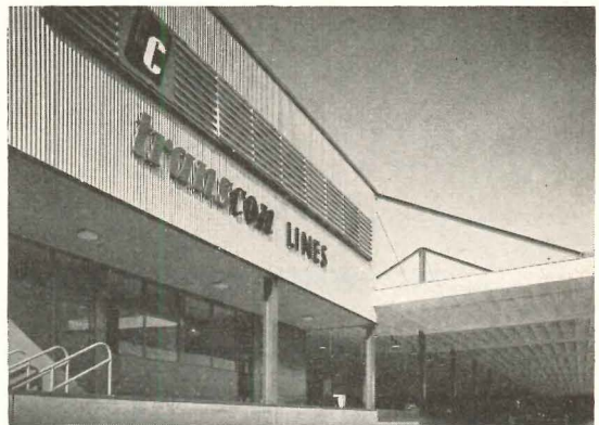
Transcon Lines, Los Angeles, p. 178. Main feature is the suspended wooden roof which has a 35-ft overhang, shielding trucks from hot sun. Two years of planning, including a tour of major terminals, helped simplify and streamline operating procedures
