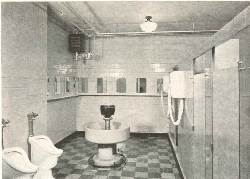
Plant walls are buff structural tile exposed on the inside; in offices and toilets walls are light green structural glazed tile. Plant floors are concrete with a three-quarter-in. pea gravel hard topping; floors in office areas are asphalt and plastic tile
