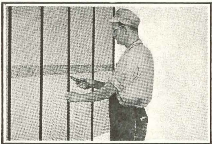
Wheeling Metal Lath ties flat to Channels with Wheeling Hank Tie Wire. Plaster is applied on both sides to form an effective solid partition.
