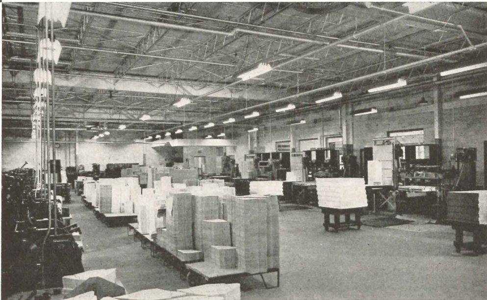
Plant walls are buff structural tile exposed on the inside; in offices and toilets walls are light green structural glazed tile. Plant floors are concrete with a three-quarter-in. pea gravel hard topping; floors in office areas are asphalt and plastic tile
