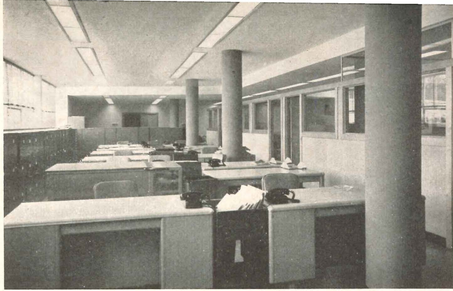
Interior trim is white birch, floors are asphalt tile, ceilings acoustical plaster. Overhead fluorescent lighting was designed to eliminate shadows, need for desk lamps
