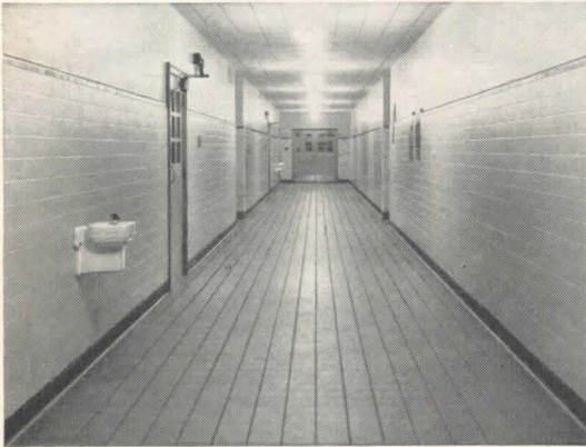
Corridor, Utica Free Academy, Utica, N.Y. Kinne & Frank, Architects.
