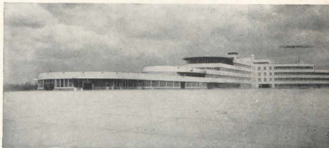
Mammoth decks in this fabulous $10-million terminal building at $42-million Greater Pittsburgh Airport, were poured on Steeltex Floor Lath. Last year 2.5-million people including travelers spent $20 million at ticket counters, restaurants, nightclub, theater, hotel and shops. Joseph Hoover, Architect. Leland Cook, Structural Engineer. Dick Construction Co., Contractors.
