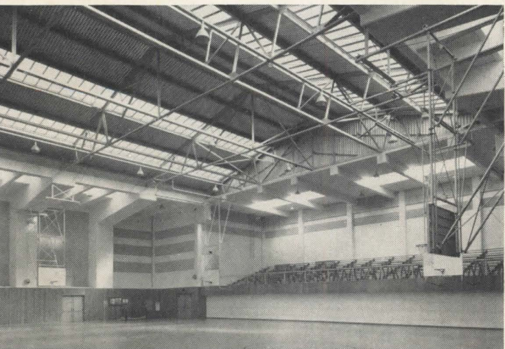
• GLARELESS OVERHEAD LIGHTING . . . There is no glare either to contestants or spectators when daylighting is handled like this. These are Robertson Corrugated Wire Glass Skylights at Herbert Hoover High School, San Diego, California.
