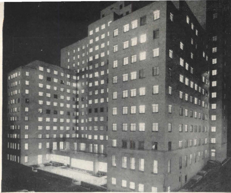
The $3.5-million nurses home at University of Pittsburgh towers 14 stories, completely air conditioned, contains library, recreation room, reception rooms, cafeteria seating 400—comfortable living quarters for 600. Steeltex in upper floors. Ingham, Boyd & Pratt, Architects. Trimble Company, Contractors.
