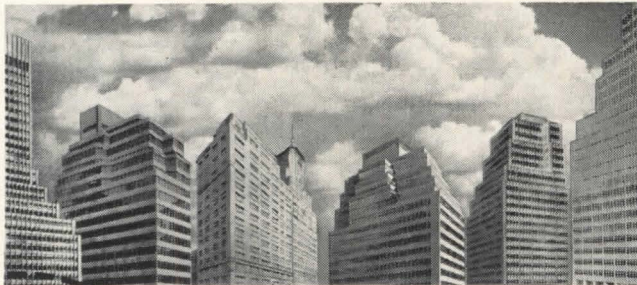
In six of New York's newest skyscrapers TRANE Custom-Air systems are installed. The Custom-Air system utilizes UniTrane room units combined with a central source of ventilation air to give complete air conditioning comfort plus individual tenant control of room temperature. Installations include 99 Park Ave.; 579-589 Fifth Ave.; 7 Park Ave.; 261 Madison Ave.; 720 Fifth Ave.; 460 Park Ave.
