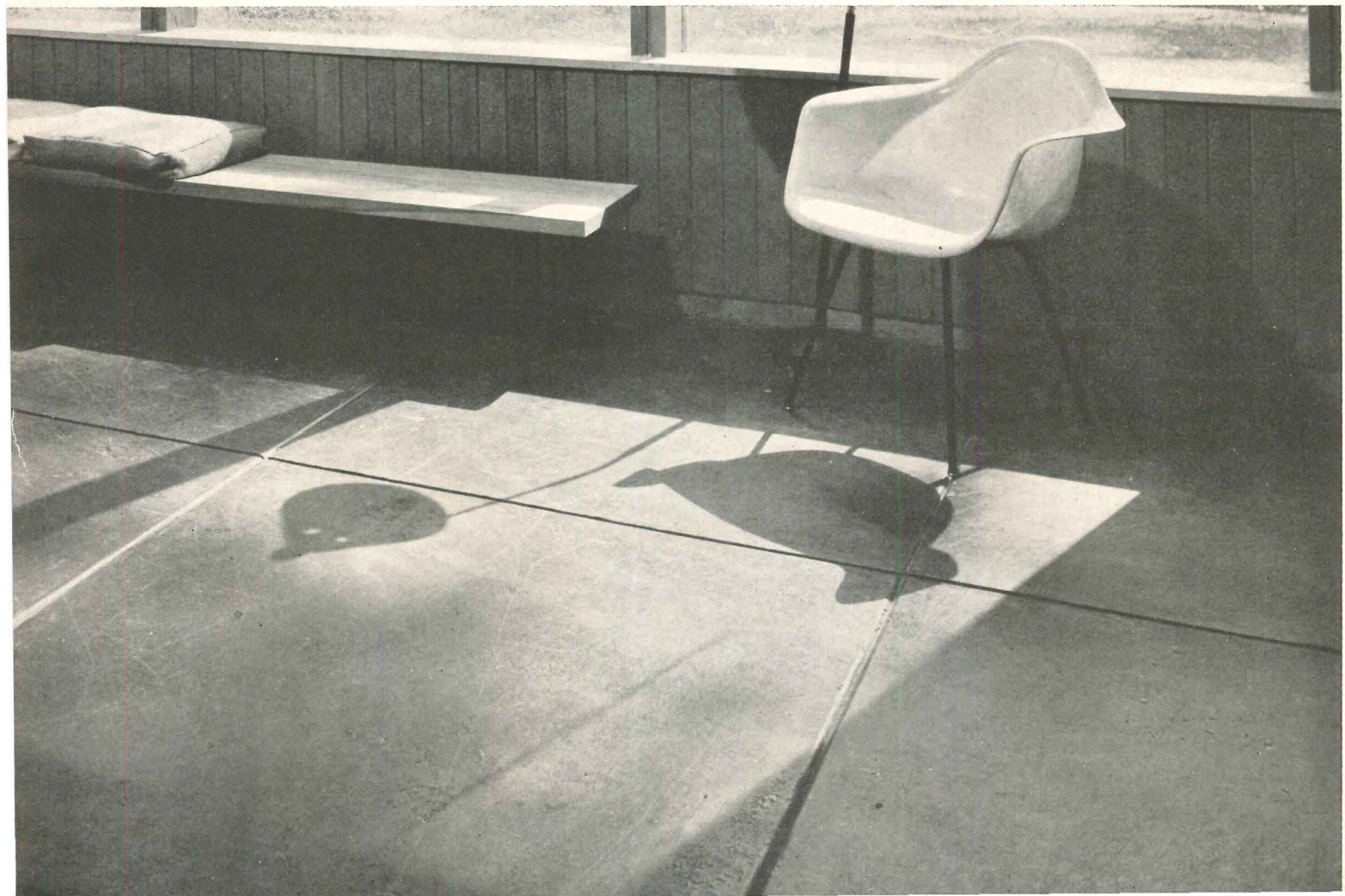
Large squares of slate: George Fred Keck - William Keck, architects. Hedrich-Blessing photo
