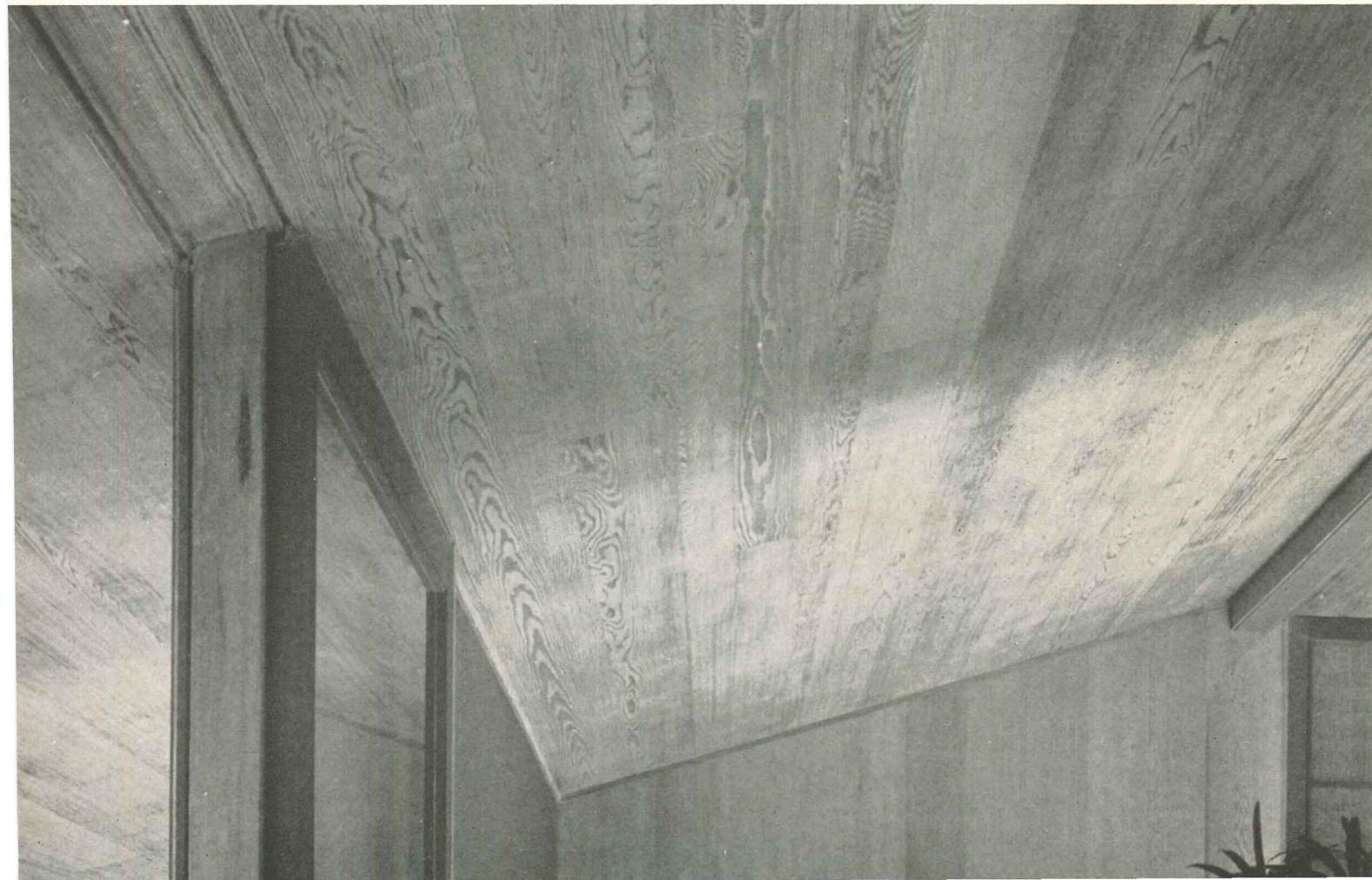
Wirebrushed redwood tongue-and-groove. Vladimir Ossipoff, architect. R. Wenkam photo
