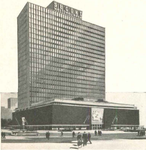
2nd National Bank Building, Houston, Texas. Architect: Kenneth Franzheim, A.I.A., Houston, Texas; Contractor: W. S. Ballows Construction Co., Houston, Texas; Aluminum: General Bronze Corporation, New York, New York.
