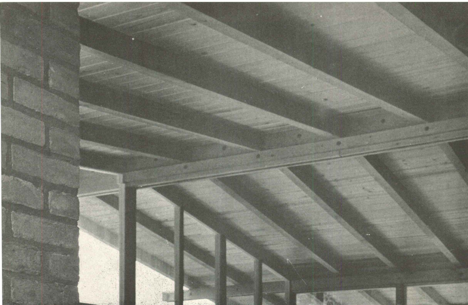
Wood beams and paneling: R. Gommel Roessner, architect. Mears Photography photo
