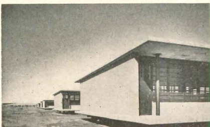
Dormitory units, Louisiana State Penitentiary
