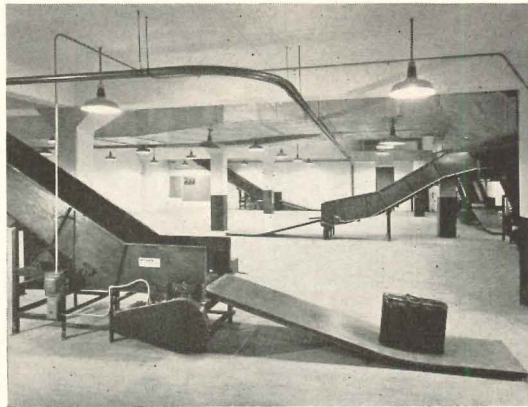
Truck ramp enters (right, photo above) finger level; trucks pick up baggage (photo below, right) from conveyors from airline counters on floor above. Emplaning passengers descend to finger level by escalators
