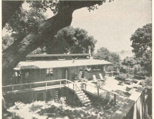
House for Mr. and Mrs. Theodore Bernardi, Sausalito, Cal. — Architects, Wurster, Bernardi & Emmons; Consulting Engineer — A. V. Saph Jr.
