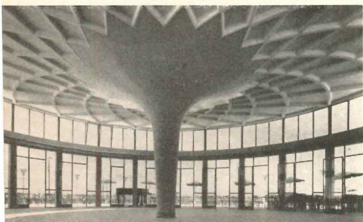
A highly expressive geometric pattern was formed in the ceiling of this restaurant designed by A. La Padula through a refinement in Nervi's pre-fabrication techniques. Precast, coffered sections, about 1-in. thick were assembled on a platform with spaces left between for reinforcing of the stiffening ribs
