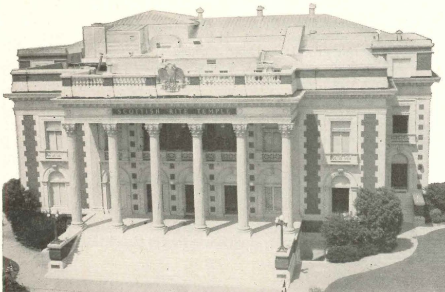
Masonic Temple, Dallas, Texas—The roof was coated with Karnak Aluminum-Asphalt Coating by Wright Waterproofing Co., Dallas
