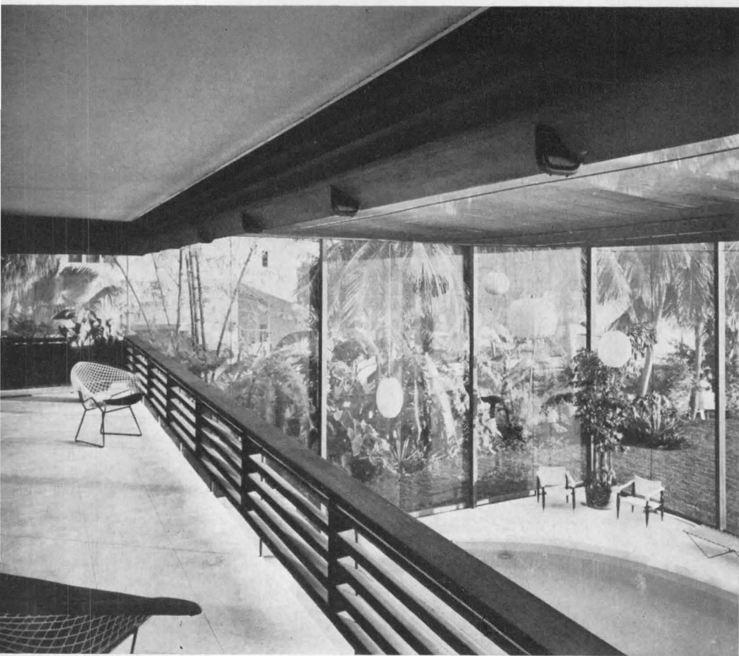
The upstairs bedrooms of the Miller house all open on the cantilevered balcony. The balcony serves as a corridor, and expands the daytime use of bedrooms as sitting areas. The lowered railings block direct view from pool area into bedrooms
