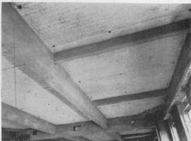
Sprayed fiber was blown on 100,000 sq ft of cellular steel flooring, giving 3-hr rating, in the Baltimore Commercial Credit Building
