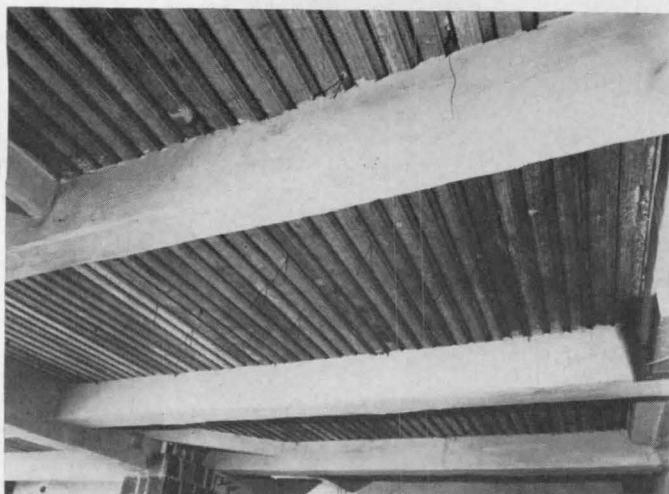
Sprayed fiber was blown on 100,000 sq ft of cellular steel flooring, giving 3-hr rating, in the Baltimore Commercial Credit Building
