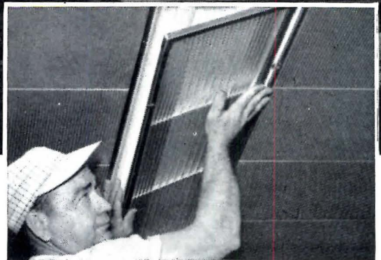
The new Kansas State Office Building is illuminated by luminaires manufactured by the WESTINGHOUSE ELECTRIC CORPORATION, Lighting Division, Cleveland, Ohio. Lenses for these fixtures (see inset) of Du Pont LUCITE acrylic resin were injection-molded by the HOLOPHANE COMPANY, INC., New York, N. Y.
