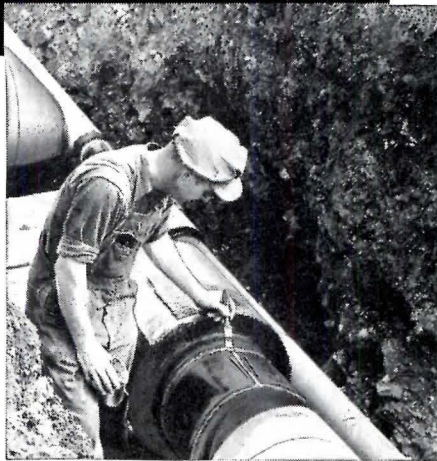
During air test, conduit field welds are checked with soap solution.
