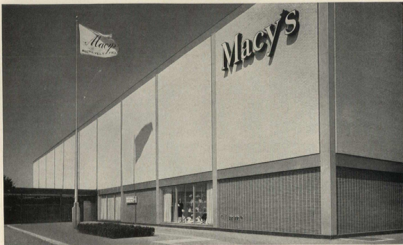
R. H. Macy & Co., Roosevelt Field, L.I., N.Y. Architects: Skidmore, Owings, and Merrill; Consulting Engineers: Syska and Hennessy, Inc.; General Contractor: Turner Construction Co.; Mechanical Contractor: J. E. Schechter Corp.
