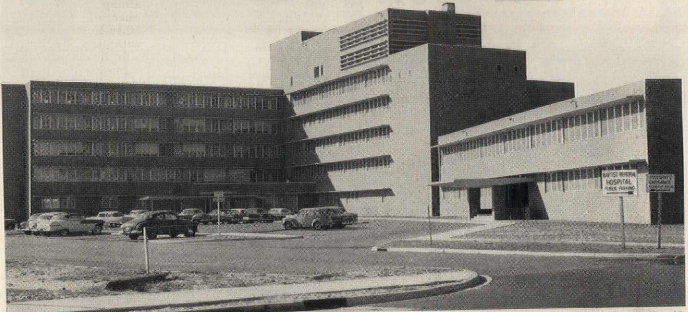
A 175 KW Cat Electric Set takes over within seconds if commercial power fails at Baptist Memorial Hospital, Jacksonville, Fla. Emer-
