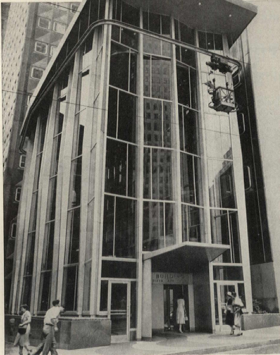
Washing windows on the inside of the lobby. The same cage is used both outside and inside.
