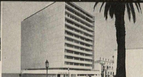
3325 Wilshire Blvd., office building, Los Angeles, Calif., uses Zonolite Plaster Fireproofing and Zonolite Spandrel Back-up System throughout. Arch.: Victor Gruen. Plast. Contr.: Martin Bros.
