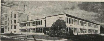
Muhlenberg Elementary School Addition - Allentown Arch.: Lange & Everett, Allentown
