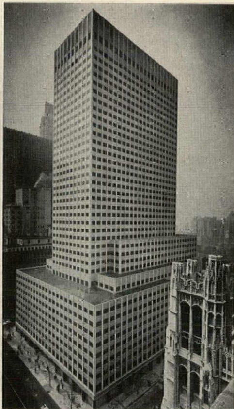
New York—666 Fifth Avenue; Tishman Realty & Construction Company, owners and builders; Carson & Lundin, Architects. New neighbor to the north of Rockefeller Center, this 38-story building has "world's largest bolted steel framework" and "world's largest aluminum curtain wall." Occupying 200 by 300 ft plot, it contains over a million sq ft of office space. Estimated cost: $40 million
