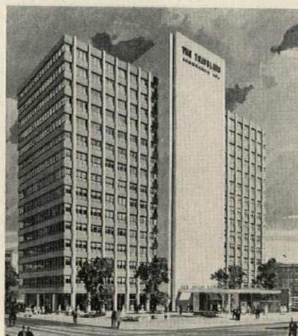
Boston—The Travelers Insurance Companies, 125 High Street; Kahn and Jacobs, Architects. The building will rise 16 stories (one more than rendering shows), its center section, housing utility core, three stories higher; it will contain 298,000 sq ft of floor area. Cost is estimated at $7 million. The Travelers tentatively plans to occupy four floors and lease 12. Structure is steel, facade blue and white brick. Building will be air conditioned
