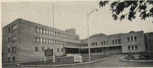
NANTICOKE STATE HOSPITAL Nanticoke, Pa. Architects: Schmitt & Lippi. General Contractor: Stan Seiple, Inc. Painting Contractor: William W. Davis Co.
