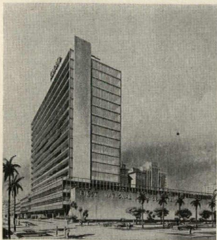
Miami—First National Bank, DuPont Plaza; Weed, Russell, Johnson Associates, Architects. The 17-story structure, scheduled for completion late this year, will provide 450,000 sq ft at estimated cost of $6 million. Bank will occupy first three floors (about 40,000 sq ft each); the other 14 floors of tower space will be rented to tenants. Structure is field-welded structural steel, facade precast concrete panels faced with ceramic tile
