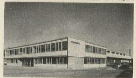
Office Building, Canadian Kenworth Trucks, North Vancouver; Semmens & Simpson, Architects. Cost: $500,000
