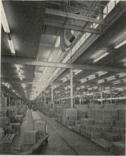
In the shipping center, two dragline conveyors transport orders. Unit ventilators are up out of the way inside the monitors
