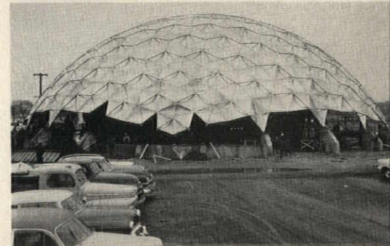
Panels are bolted in place
