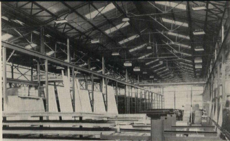
Infrared generators—sans ducts, blowers and heat exchangers—maintain even temperature, dispel damp
