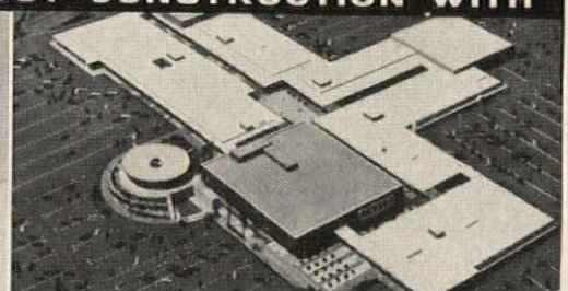
Gulfgate Shopping City, Houston, Texas, has Zonolite Plaster Fireproofing throughout. Arch.: John Graham & Co. Plast. Contr.: Tobin & Rooney.
