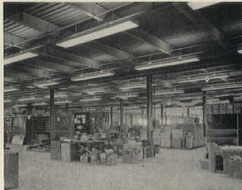
"BI-FLO UPLIFTER" 72% downlight — 28% uplight, provides greater seeing comfort for industrial areas such as Assembly Lines .
