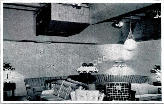
General Electric Celling-Mounted Units at the Dailas Home Furnishings Mart take no floor space —provide Individual temperature control (heat and cool)—are metered for zone control of operating cost.
