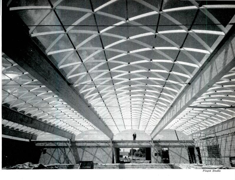
rises above the surrounding building, and provides a clerestory with vertical louvers. Continuous plugin strips will be placed along the bottoms of the beams to give maximum flexibility for lighting.
