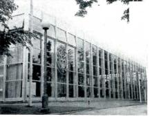
Fabricated in Italy, the large building is steel with three walls of glass supported by vertical aluminum frame members; the other wall is of asbestos paneling. Unobstructed exhibit space is achieved by means of welded tubular steel trusses fastened to round steel columns on the perimeter. The concrete floor slab is laid over electrical ducts. The building is 170 ft long, 95 ft wide, and 32 ft high.
