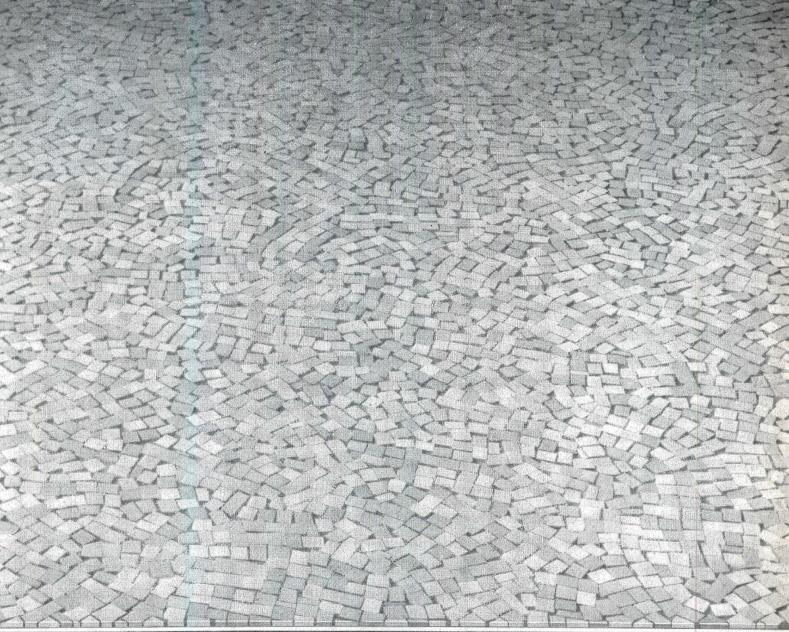
Color chips are actual size in foreground of photo. Translucent vinyl grouting gives three-dimensional look to an actually smooth surface. White line beneath chips is alkali-resistant Armstrong Hydrocord Back.
