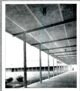
Weather-resistant, good-looking INSULROCK used as roof decking provides ceiling for corridor outside classrooms of new Hillcrest High School, Simpsonville, S. C. Architect: Wm. Freeman & Associates; Contractor: Triangle Construction Company, both Greenville, S. C.
