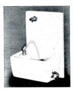
No. 5623—Streamlined face-mounted drinking fountain, heavy vitreous china, integral trap housing, concealed well hanger. Two-stream mound-building projector and Halsey Taylor automatic stream control.
