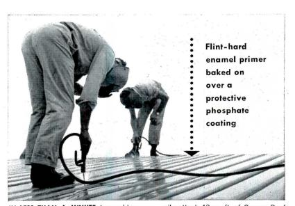
IN LESS THAN A MINUTE, two welders can easily attach 43 sq. ft. of Granco Roof Deck to framing. Wide-cover sheets mean fewer laps and welds. Long sheets (up to 211/2') permit continuous spans, greater economy. Strong sheets provide better support for heavy loads. And look at the finish! Smooth, tough, tightly bonded to Granco steel. Enamel is "flo-coated" over steel and baked on at 350° F. for 20 minutes. No roof deck on the market is better protected against abrasion and corrosion!
