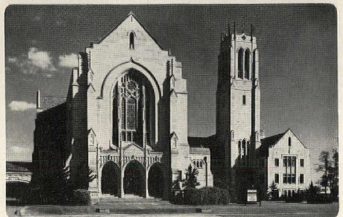
St. Paul's Methodist Church in Houston, one of the finest in the City, is air conditioned with Frick "ECLIPSE" compressors.
