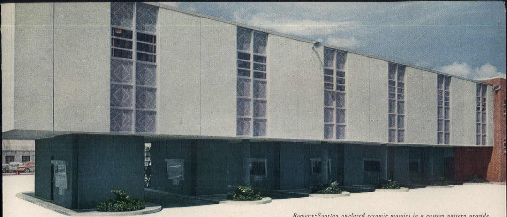
Romany•Spartan unglazed ceramic mosaics in a custom pattern provide the exterior wall finish for Orlando's new Citizens National Bank.
