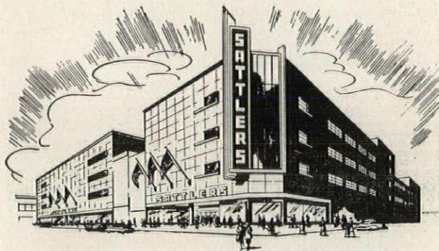
Sattler's was the first completely air conditioned department store in Buffalo—has used Frick equipment since 1937. Sattler's Annex is cooled with 21 Frick unit conditioners.
