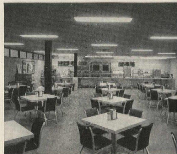
Cafeteria in the headquarters building in the service and supply area. Here flush mounted troffers with curved lenses assured a pleasing lighting effect of low brightness luminescence.
