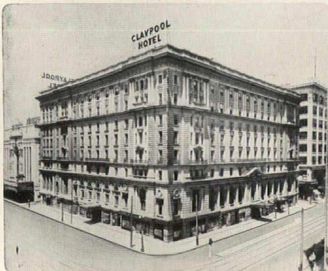
The Claypool at Indianapolis is said to be the first large hotel in the North completely air conditioned. "ECLIPSE" compressors carry the cooling load. The Hotel has used Frick refrigeration for food service since 1939.
