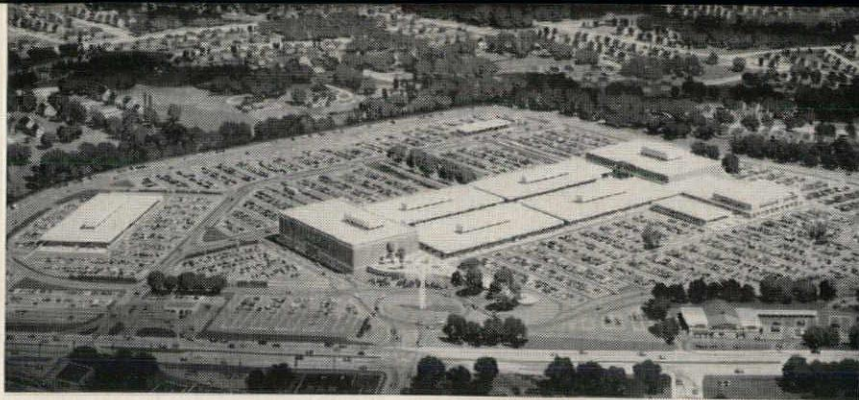
The Wheaton Plaza Regional Shopping Center, Wheaton, Maryland Arthur L. Anderson, Architect. Lathrop Douglass, Consulting Architect J. Gibson Wilson, Jr., and Beall & LeMay, Consulting Engineers
