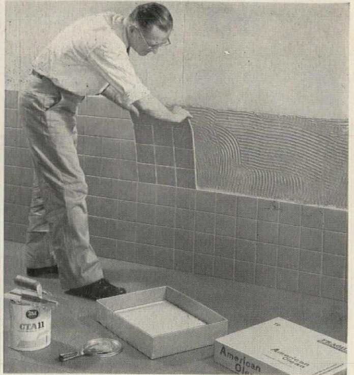
Master-Set sheets go from carton to wall in one motion with no soaking needed—can be installed with adhesives, thin-set mortar, or conventional cement mortar with self-curing bond coat.
