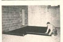
**SISALKRAFT**, tough, reinforced waterproof papers for protecting floors, curing concrete, covering unfinished work on the job. In fact, any application requiring protection against the weather.
