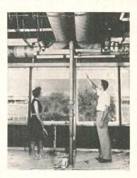
School Heating, Ventilating System A new method for heating and ventilating schools will reduce costs by as much as ten per cent, according to the manufacturer. Working on the principle of high velocity induction, the system is similar to the forced warm air systems commonly found in homes but differs from them in that more air is circulated and each outlet contains a coil for reheating room air induced through it. The reheat coil acts like a baseboard con-
