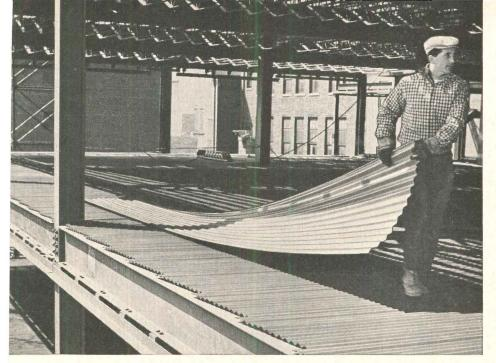
Extra-long lengths of coated Fab-Form, 27 feet, 3 inches, were specially commended by job superintendent on Looman Building job. "Fab-Form's extra-long length and wider width certainly helped to get these floors and roof poured faster," he declared. "I'm convinced the red oxide finish has better corrosion resistance than other coated sheet material."
