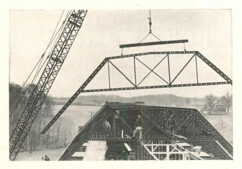
After fabrication, roof trusses were raised into position by a mobile crane and securely welded in place in a matter of minutes. Smaller panels were light enough to be carried and erected without handling equipment.
