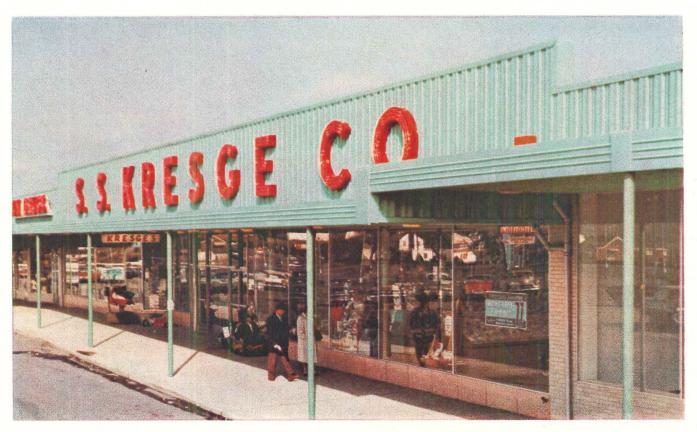
In this new shopping center, building facing, as well as canopy soffet are EGSCO Shadowall Panels. Color is baked-on epoxy enamel. Canopy facia was specially formed of the same durable metal and color.
