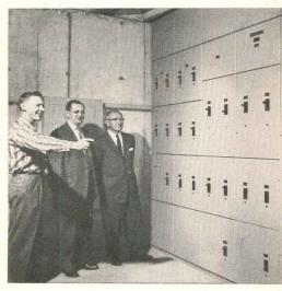
A. J. Eversmann, Maintenance Superintendent of WAVE, inspects the modern and compact Westinghouse building-type switchboard with R. A. Schlaug and M. D. Bornstein, both of Bornstein Electric Company. Westinghouse AB De-ion® circuit breakers distribute and protect all power circuits in the studio. Provision is made to install additional breakers when required in the future.
