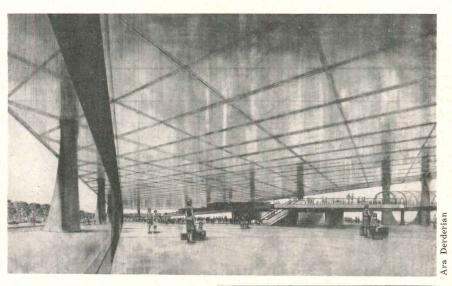
Pei's city-block-long rectangular structure is encased on four sides with glass walls. Two-story-high concourse runs full length of the building. Ticketing and baggage counters are on first floor; waiting areas and shops are on island-like mezzanine. Vehicular roadway gives access to both front and field side of building. Passenger arcades to aircraft are bridged over road on field side, which is separated from aircraft apron by fencing
