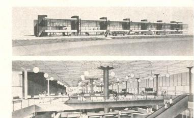
Morris Ketchum, Jr., Ketchum and Sharp: stairwells divide building into 7 glass-walled sections. Columns support concrete roof with radiating roof structure
