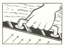
6. Final troweling compacts the surface, leaves it smooth. The trowel produces a ringing sound but not as noticeable as with regular mixes.
