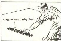
4. Delay wood floating for 30 to 40 minutes after the concrete is placed. If stickiness appears when wood floating is started substitute a magnesium darby float—use sparingly and in a flatter position than for regular mixes.
