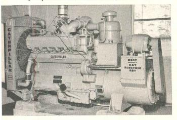
Cat D326 Diesel Electric Set is used for standby power at Water Department in Warren, Ohio.
