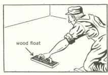
4-a. If the wood float is used, steel trowel sparingly in about 10 to 20 minutes after the wood floating is completed. Don't overtrowel. If stickiness appears, delay troweling for 15 or 20 minutes or until stickiness disappears.
