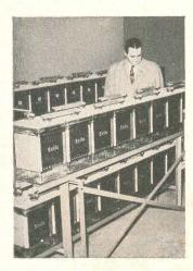
Emergency power source Powerful Exide Batteries can handle lighting loads for entire buildings. Long service life up to 25 years is common.
