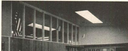
Above: With glass transoms, reflections of fixtures, as well as view of fixtures in adjacent rooms, can be easily avoided by positioning primary light sources below the level of the glass. Right: The lack of specular or fixture reflections on the glass adds elegance to this canopied entrance. Far right: sketches show various methods of preventing reflections of light sources in polished materials—mirrors, glass and marble
