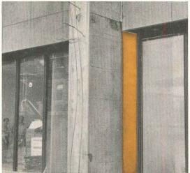
UPRIGHT CONCRETE GIRDER before covering with bronze "skin." The Revere Muntz Metal used was in thicknesses of 1/2" and 3/16", ranging up to 40" in width by 11' 11" in length.
