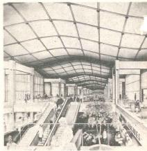
Philip Johnson, Philip Johnson Associates: undulating roof is made of grid of steel pipes which support precast concrete roof planks. Structure front has lower stone facing, upper decorative grille
