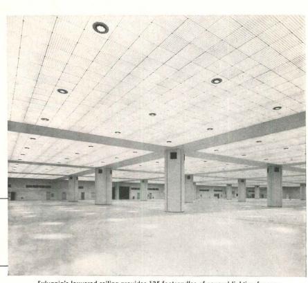
Sylvania's louvered ceiling provides 135 footcandles of general lighting for over 100,000 square feet of display area. Complete system consists of outrigger-type fixtures with eight 75-watt Instant Start lamps installed in a grid arrangement.
