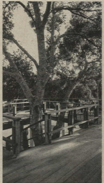
The all-heartwood grades of redwood are ideal for terrace decking as they offer exceptional resistance to decay and weathering.
