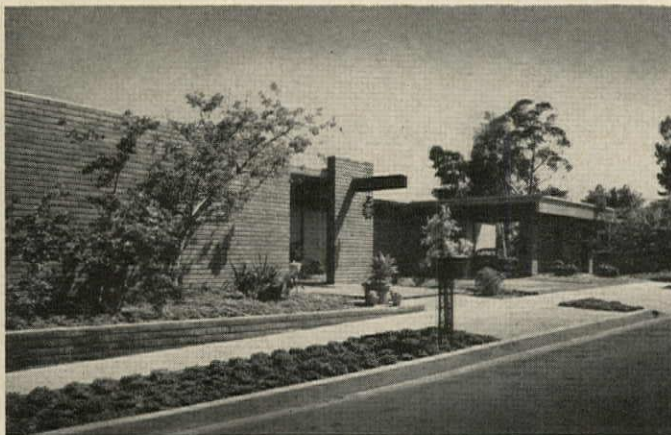
Buff, Straub & Hensman: Van de Kamp Residence for Mr. and Mrs. Walter Van de Kamp, Los Angeles. Contractor: Hugh Gates
