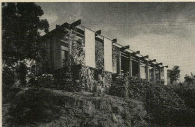
Killingsworth, Brady and Smith & Associates: Robertson Residence for John Robertson, Laguna Beach, Calif. Contractor: John Halas
