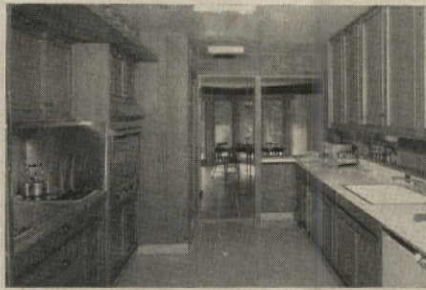
Redwood was also specified for the kitchen, including the cupboard doors. Note the insert panels of vertical grain redwood plywood, an interesting detail.
