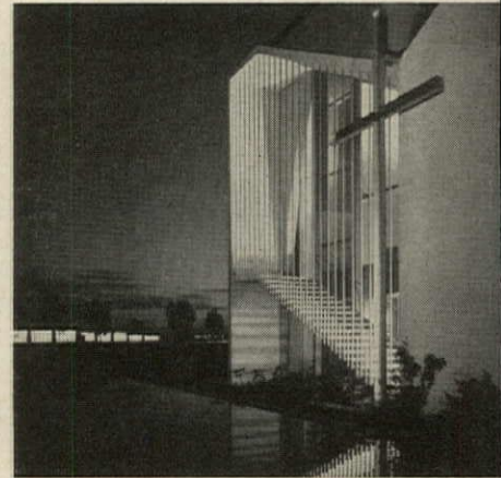
Richard J. Neutra, Robert E. Alexander, Chapel, U.S. Naval Air Station, Miramar, Calif. Contractor: Alan Rogers
