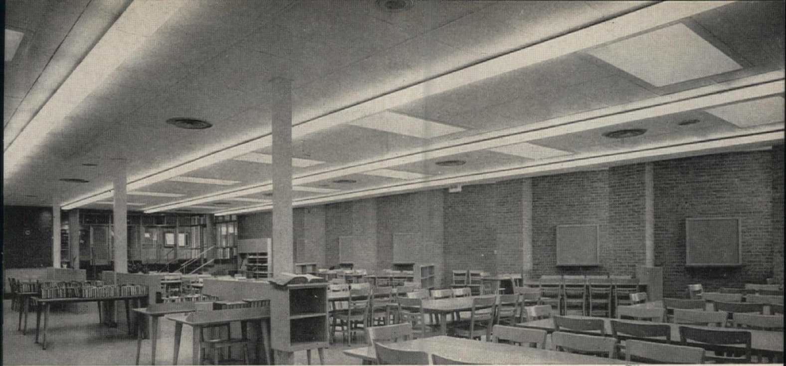
Superb Day-Brite Holiday fixtures maintain a minimum lighting level of 70 footcandles.
