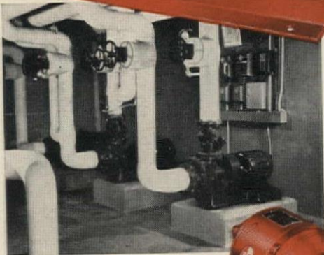
B&G Universal Pumps circulating primary mains.
