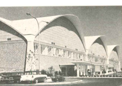
Light-controlling Thinlite panels provide excellent natural light, help reduce heating and cooling costs for the new $20-million Intelce Systems Post Office in Providence, R. I. Charles A. Maguire & Assoc., Providence, supervised design and construction.
