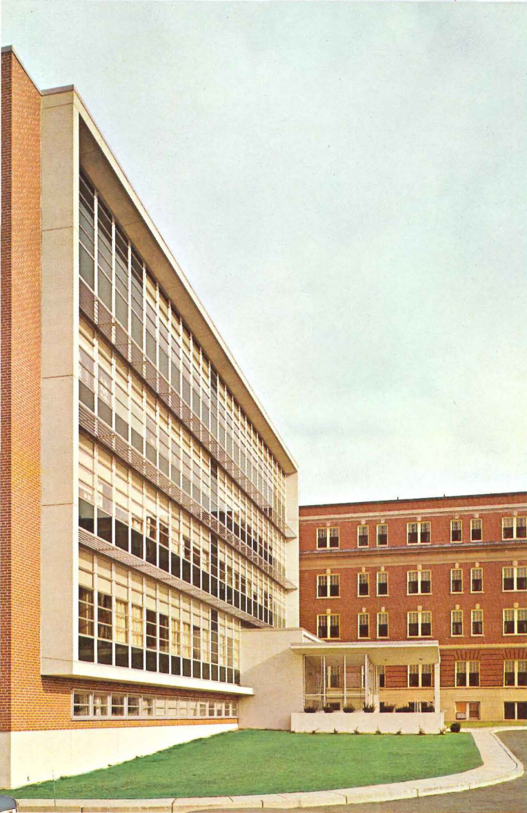
Sweeping glass façade in the new wing of Roger Williams General Hospital, Providence, R.I. Architects: Howe & Prout, Providence. L·O·F Vitrolux was used in the spandrels, Thermopane in the windows.
