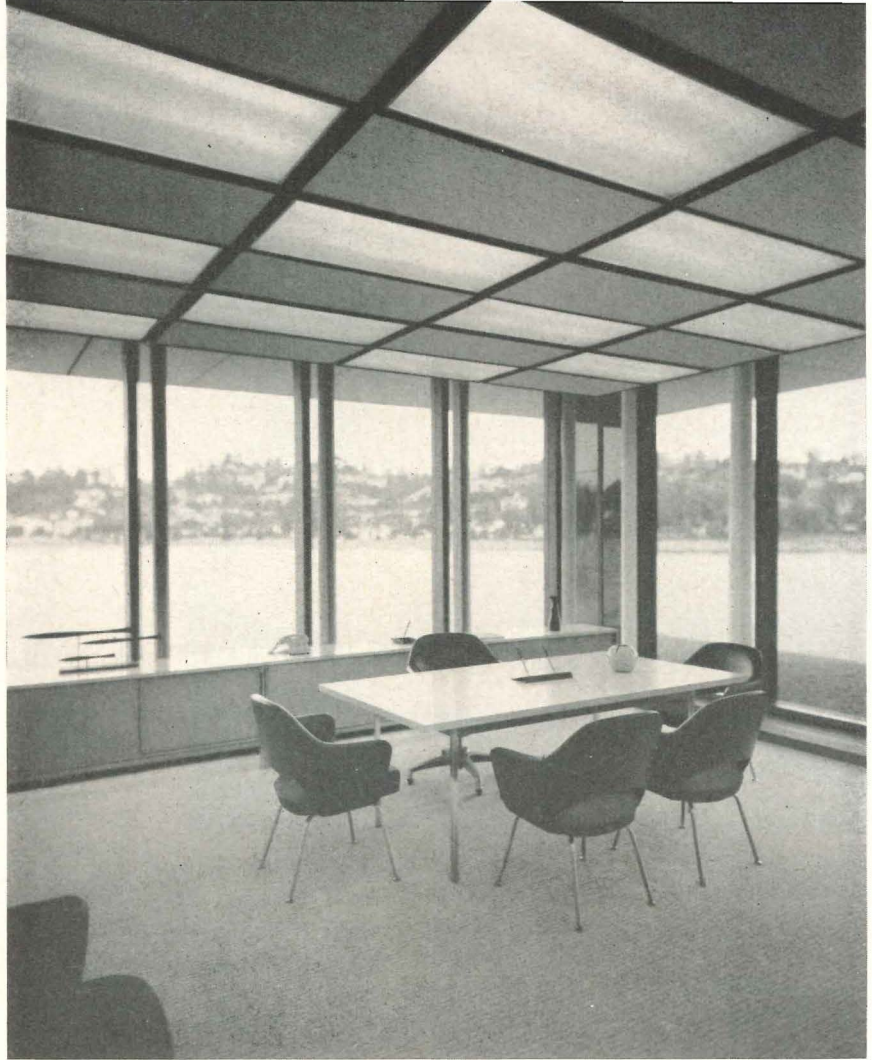
Interior of 1500-sq ft mock-up shows checkerboard pattern of ceiling which combines lighting, air conditioning and acoustical functions. Supply air issues from slots along the sides of the lighting fixtures; exhaust air is returned at one end of the fixture, passing over fluorescent tubes and into the ceiling plenum (see details below). Plenum air is used by induction boxes to temper supply air
