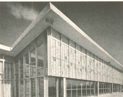
Northwest Suburban Y.M.C.A., Des Plaines, Illinois, is one of a series of new Y.M.C.A. buildings in the Chicago area in which Thinlite is used. Y.M.C.A. architect Eugene White commissioned Eckroth, Martorana & Eckroth, Chicago, to design Des Plaines Y.M.C.A.
