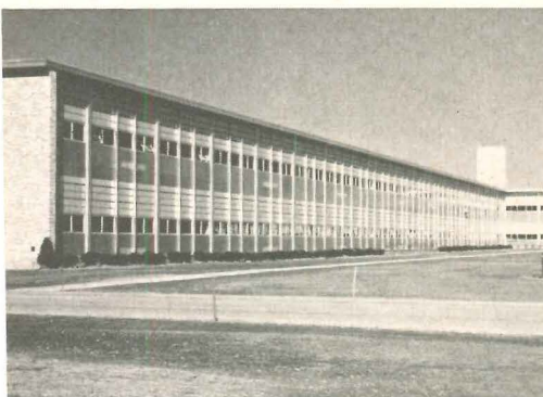
Architect Enos Cooke, New Kensington, Pa., used Thinlite in a major way at Stewart Junior High School, Lower Burrell Township, Pa., blending light-controlling panels with windows and aluminum-faced insulating panels.
