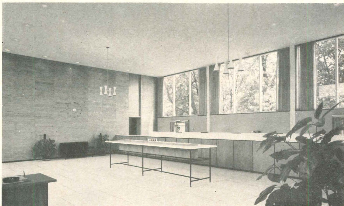
Photos by Bill Engdahl, Hedrich-Blessing
