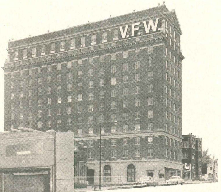
VFW BUILDING, KANSAS CITY, MISSOURI
