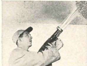
Applied in one operation. K & M SPRAYED "LIMPET" ASBESTOS combines in mid-air with water from special spray gun.
