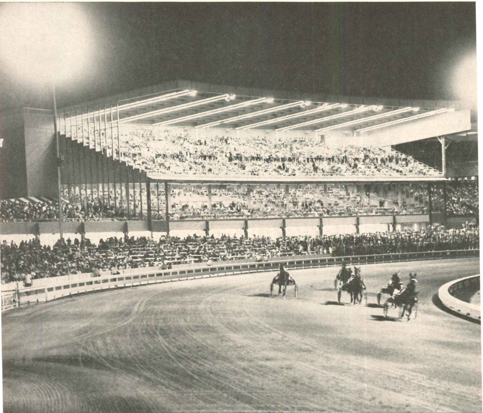
CLUBHOUSE, YONKERS RACEWAY, YONKERS, N. Y. Architect: Lionel K. Levy Roofing Contractor: Munder-Sobel & Kraus Corp. Ruberoid Specifications: Special Bitumen Spec. 202A, 203A
