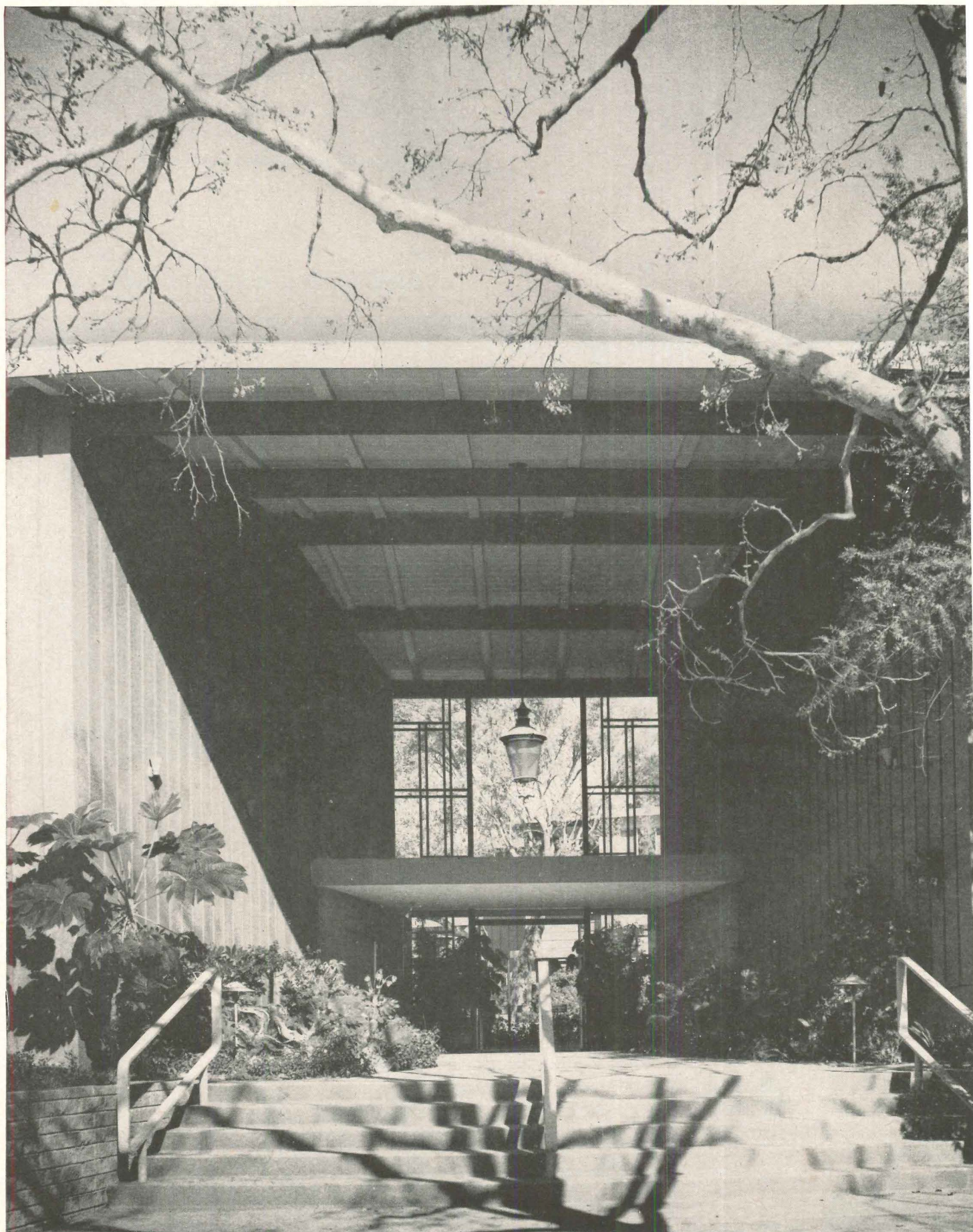
A glass-walled entrance framed with vertically channeled siding and a plank-and-beam overhead creates an imposing approach to the interior court of the Bay Tree Apartments. This extraordinary 7-unit, 2-story design is located in Los Gatos, California. Architect: Fred Marburg.
