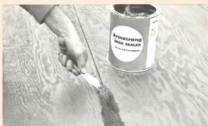
Armstrong Deck Sealer —an elastic caulking compound used in preparing the roof deck for the application of the F/A Roofing System (i.e., filling depressions, cracks, and voids in the roof deck and at joints and flashing points).
