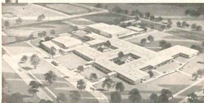
From top: Colon High School, Colon, Mich.; Augusta High School, Galesburg, Mich.; Lakeview High School, Battle Creek, Mich. ARCHITECT: Guido A. Binda, Architect and Associates, Battle Creek, Mich. MECHANICAL CONTRACTOR: Hunter-Prell, Battle Creek, Mich.
