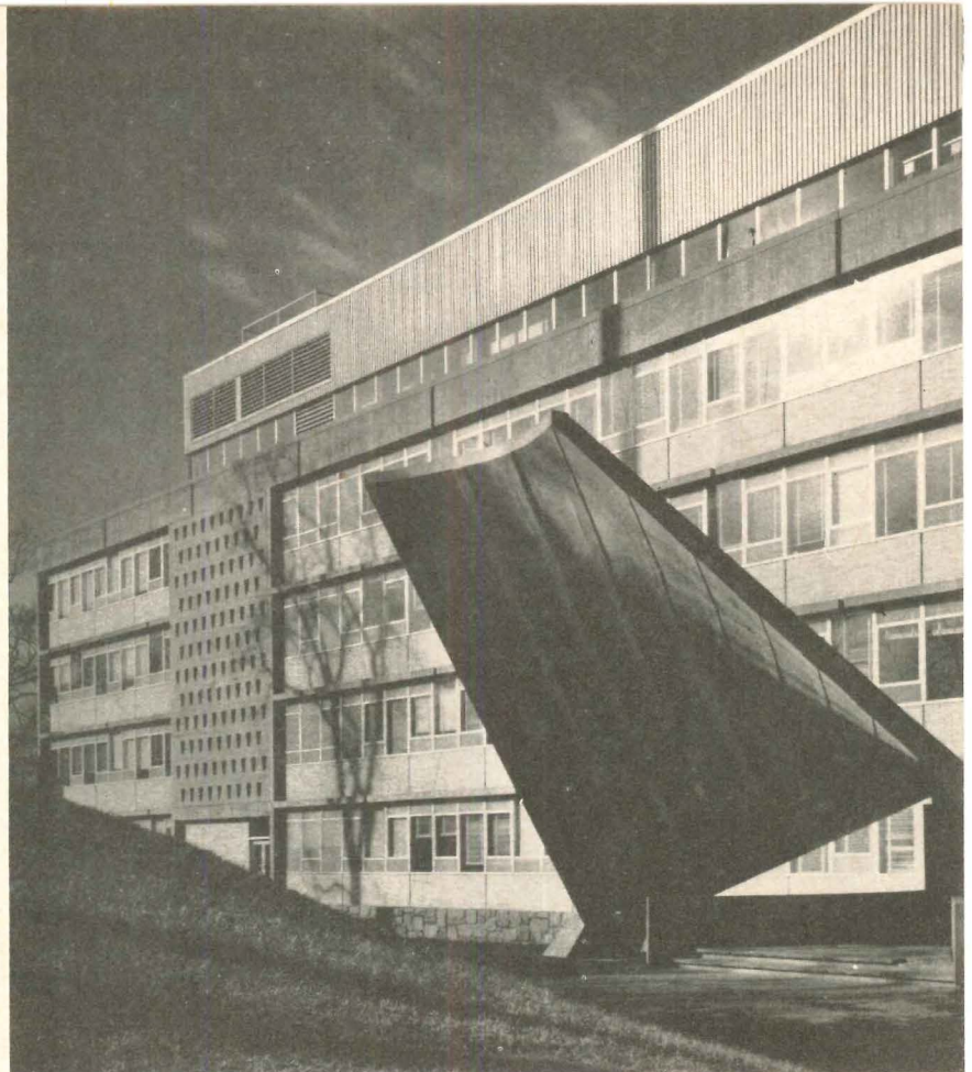
Entrance to laboratory wing on the campus side is a curved concrete canopy of thin shell construction in the saddle form of a hyperbolic paraboloid
