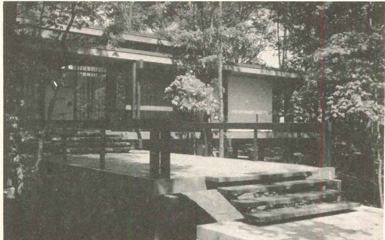
Lapierre Residence, St. Catherines, Ont. Architect: James E. Secord and Saul Herzog
