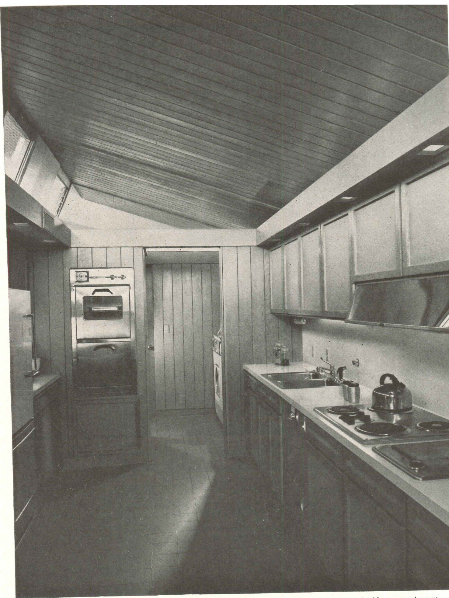
The last word in kitchens gets the right word from wood, with tongue and groove ceiling and walls, wood cupboards above and below the counters—all cheerfully brightened by well-placed windows and wood-encased cove lighting overhead.
