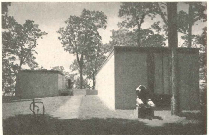
PHOTOS: © EZRA STOLLER
