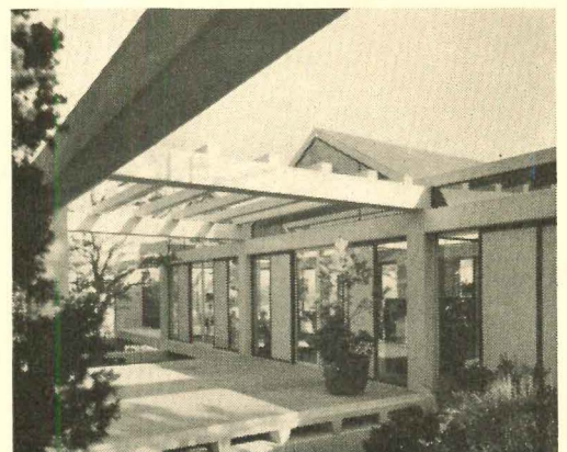
Broad entrance terrace, formed by one of the basic “Space Frame” units. Floor is of 2' x 16' precast concrete panels.
