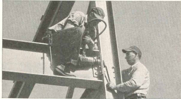
SAVE CONSTRUCTION TIME with Republic's New Heavy Head High Strength Bolt Assemblies. Two-man team replaces costly erection crews. When wrenched up tight, Republic High Strength Bolts provide a vise-like clamping force which transfers loads by friction to the structural members. Fatigue life is improved. Joints are stronger than connections where loads are carried in shear. Send coupon for illustrated folder.
