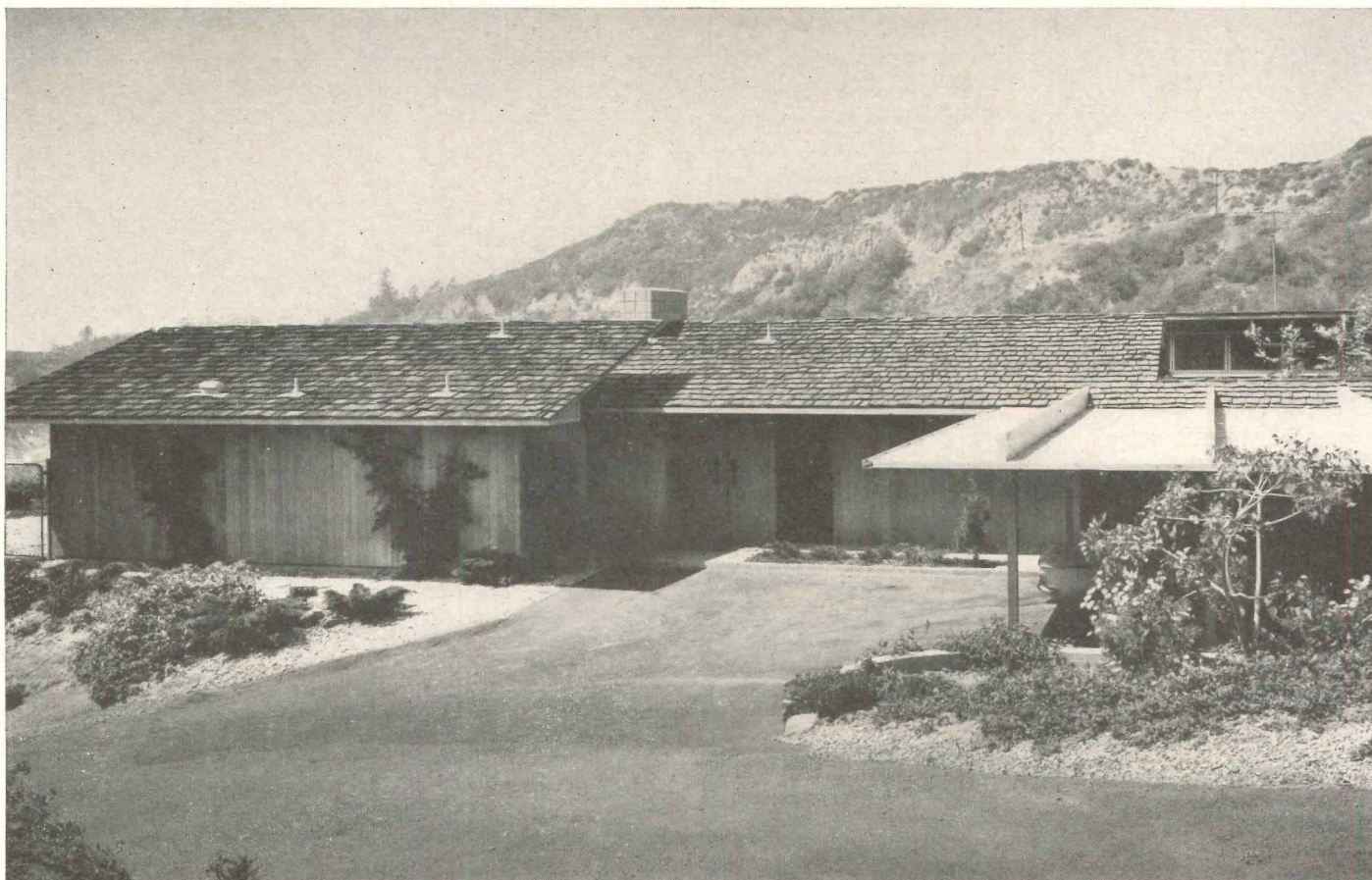
Snug in its sloping site, this contemporary's shingled roof and planked siding demonstrate some of wood's natural hillside manner. Note how the beauty of weathered wood suits this low, rambling residence designed by Rex Lotery, A.I.A., architect.
