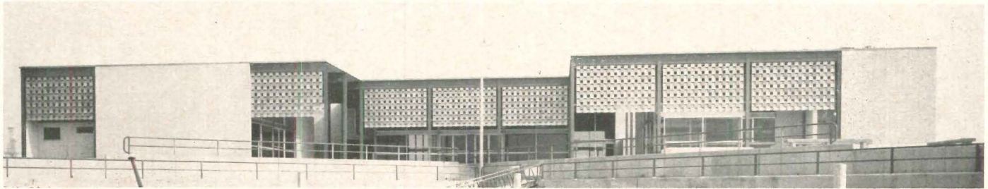
Marine Bazaar in Long Beach, California uses hard anodic coatings for aluminum columns, wall framing members and for sun-screen. Architects, George M. Montierth and Jack J. Strickland
