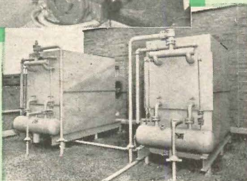
ABOVE — Two Vilter R-22 Uni-Chillers air condition Deaconess Hospital's new addition and have been cross-connected to an earlier purchased Uni-Chiller to provide an integrated, flexible air conditioning system.
