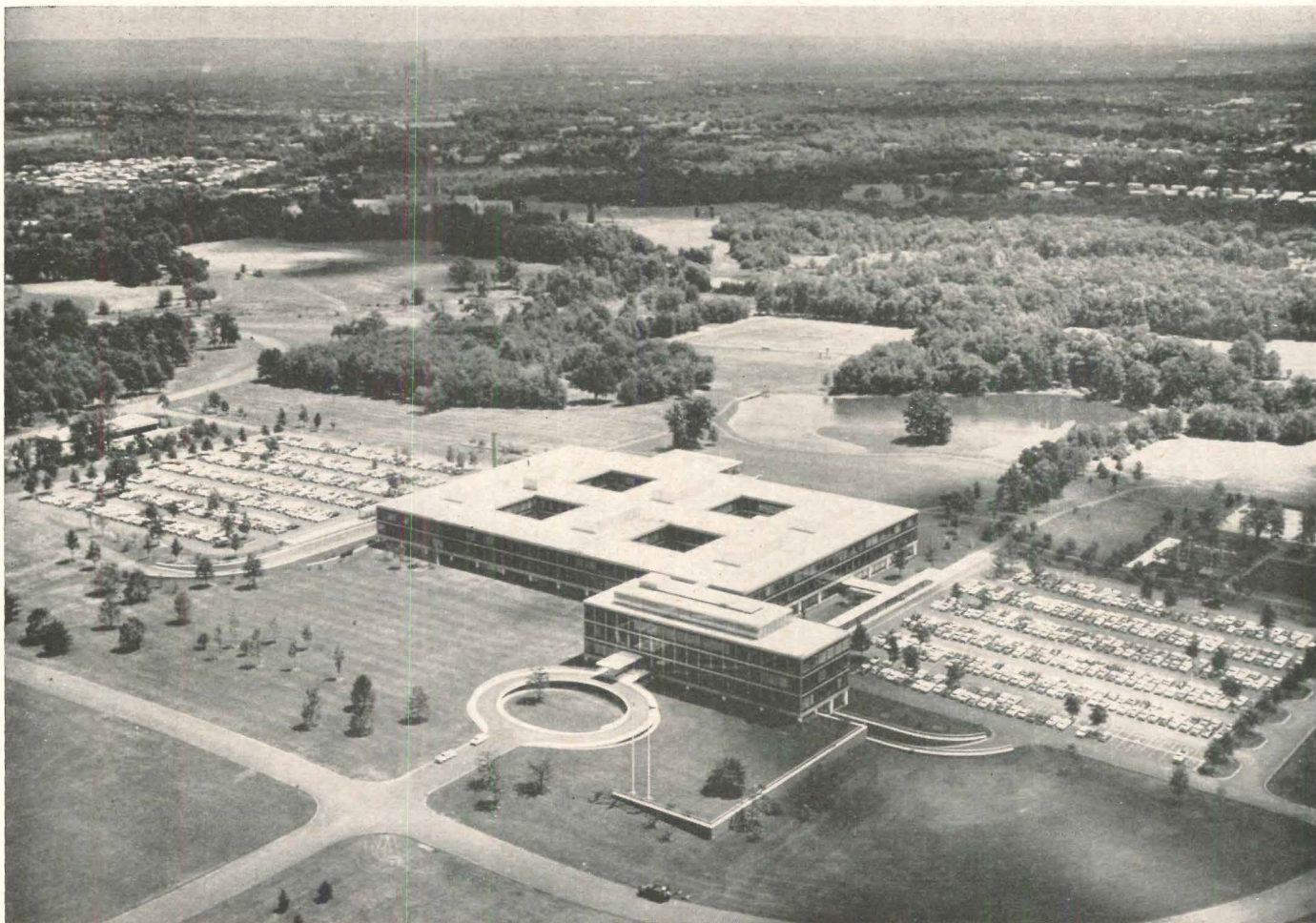
Connecticut General Life Insurance Company headquarters outside Hartford, Conn. Architects, Skidmore, Owings & Merrill
