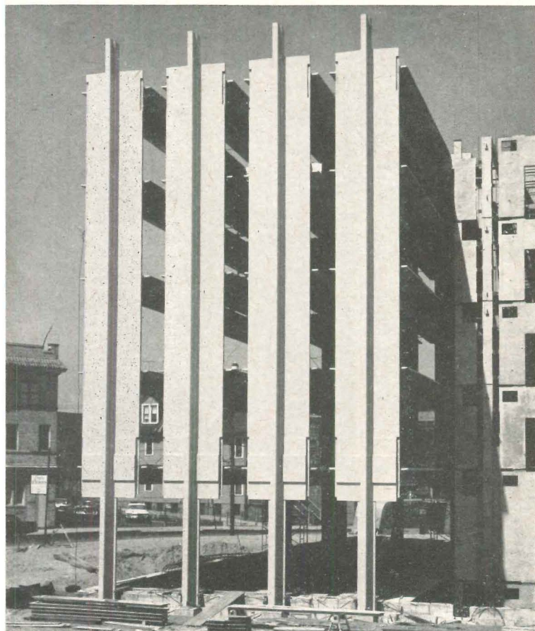
Webs of the wall-column tees, extended at the top to engage future two-story column extensions, make interesting pattern
