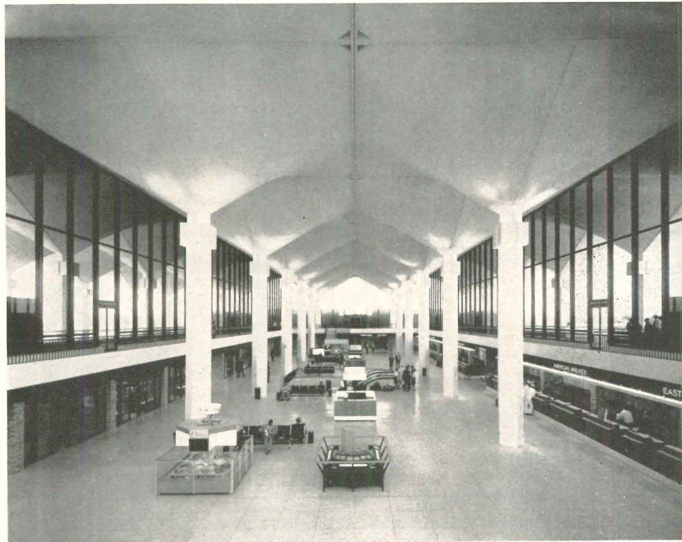
Main passenger floor as seen from mezzanine, showing hyperbolic paraboloid roof
