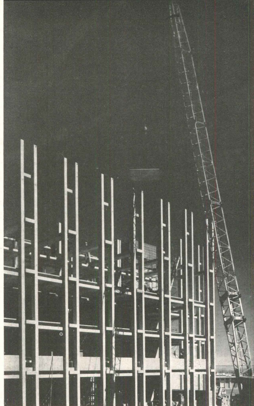
Above: Crane hoisting precast floor plank to an upper story. Some of the precast spandrels are installed. Space above the spandrels is clear glass; slot below is of tinted glass, which helps give a lighter feeling to the structure inside and out. Below: Several floor planks have been laid on beams
