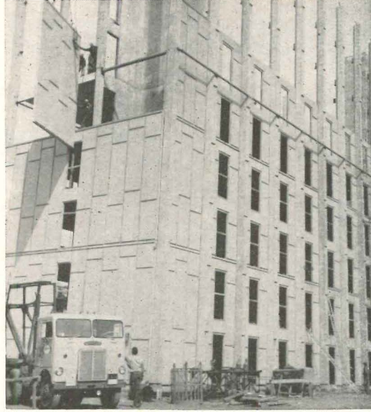
Prestressed channels span 36 ft; are supported by inverted T's set in columns. Pipes and straps temporarily brace columns
