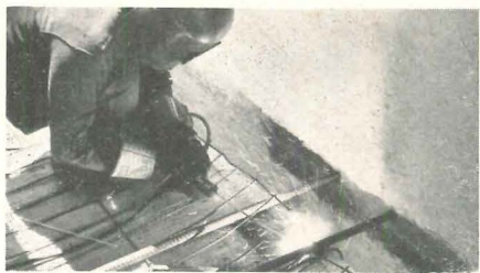
Welder making top moment connection between column tee and floor tee
