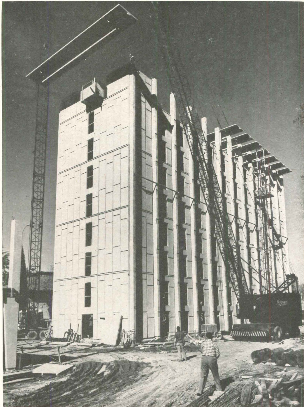
Two-story-high wall panels have grooves to provide shadow-line pattern. Roof structure consists of sculptured T-beams
