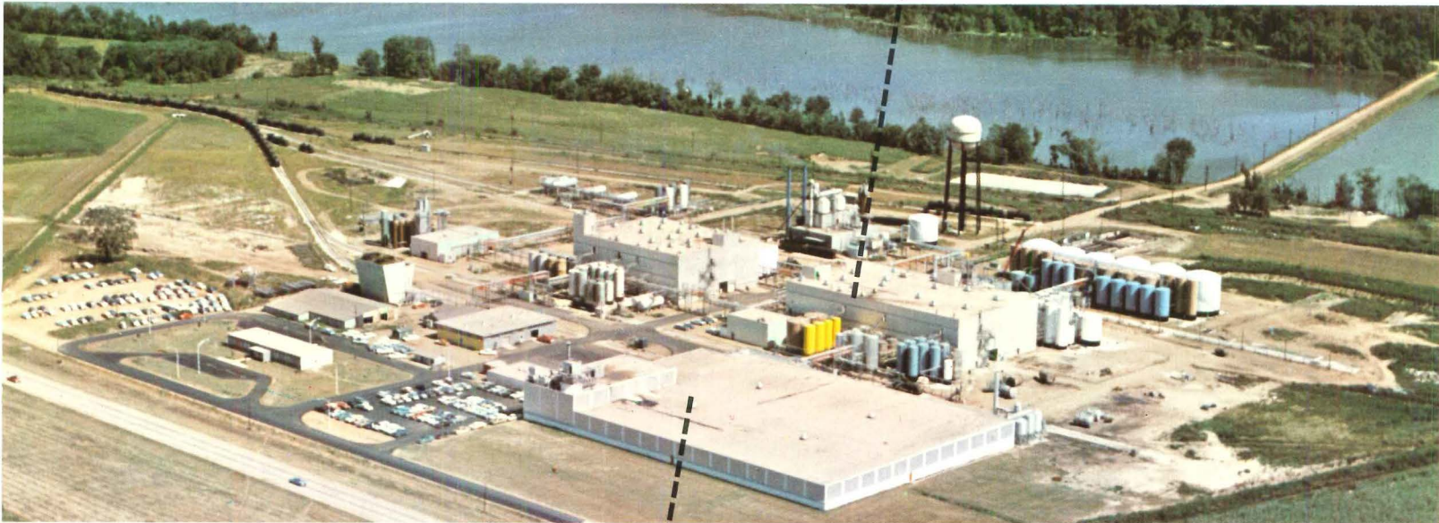
Archer Daniels Midland Company Plant, Mapleton, Illinois Designed and Constructed by Girdler Corporation, Louisville, Kentucky
