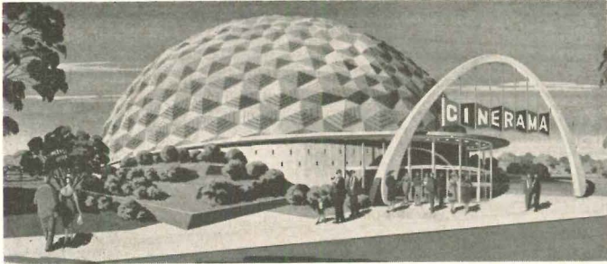
Exterior of geodesic dome movie theater using precast concrete panels with ridged pattern
