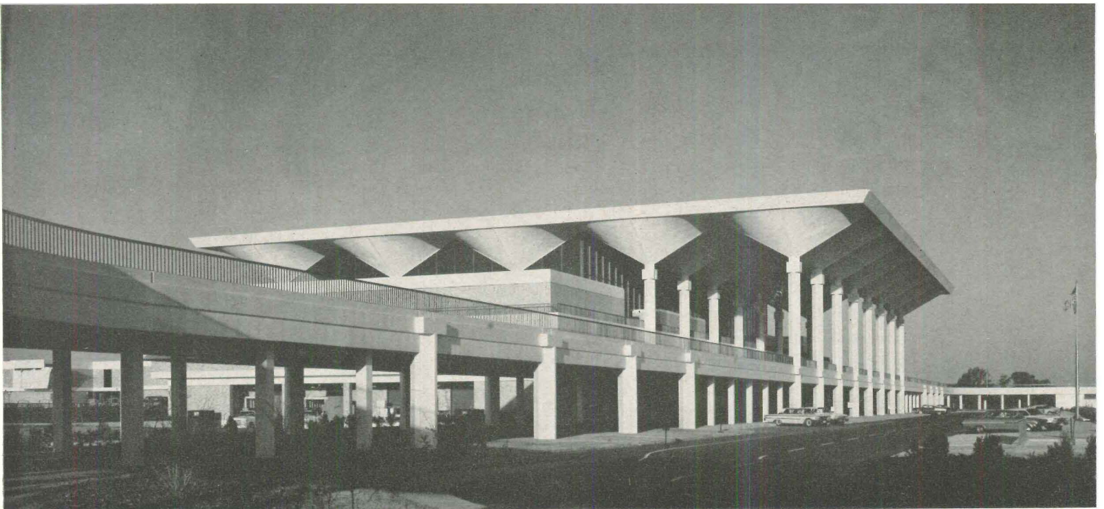
Main approach. Entrance from ramp leads to main passenger floor
