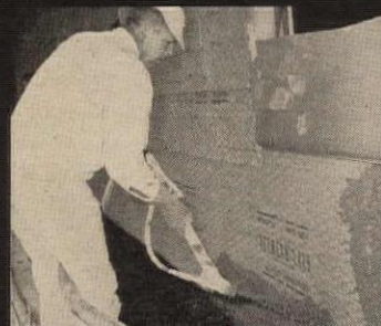
Cement trowelled prior to application of finish coat.
