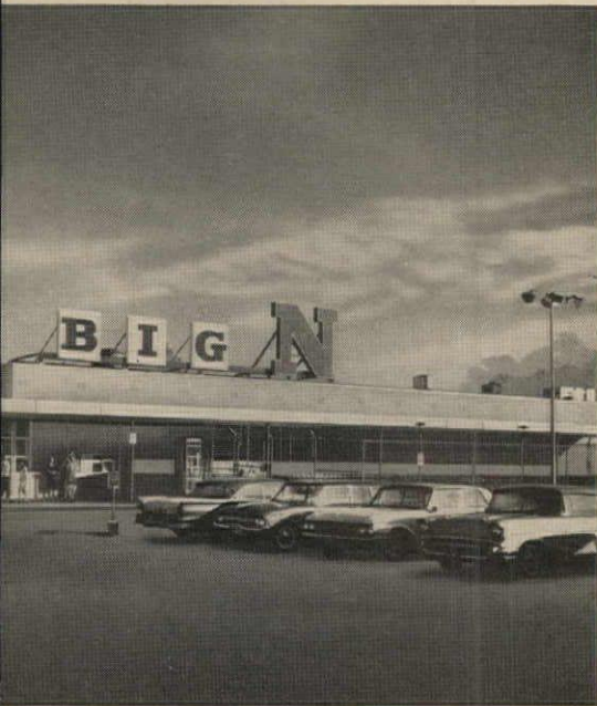
Neisner's Store, Batavia, New York, is heated and cooled by 6 York SUNLINE Air Conditioners. Conditioned air is distributed through ceiling diffusers.
