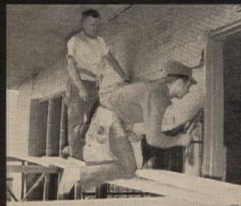
Portland Cement is sprayed on.
