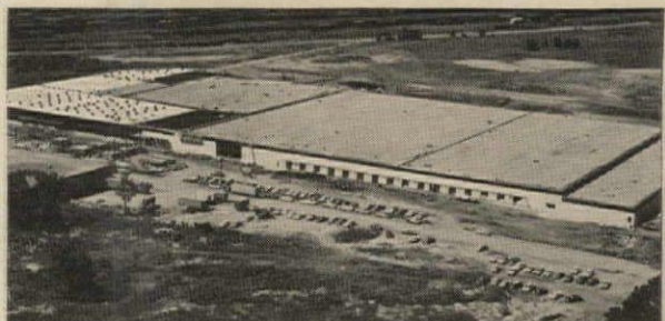
Aerial view of new Montgomery Ward warehouse in Franklin Park, Ill., Roofer: E. W. Olson Co. Engineer and Builder: The Austin Co.
