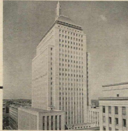
John Hancock Mutual Life Ins. Co., Boston Cram and Ferguson (Hoyle, Doran & Berry), Architects & Engineers Turner Construction Company, Builders
