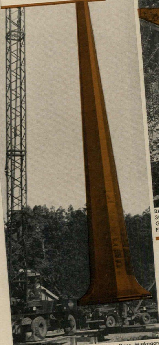
COPPER SPIRE for Church of the Open Door, Muskegon, Mich. It was fabricated from 5,000 lbs. of 16 oz. Cold Rolled Revere Copper by LIVINGSTON SHEET METAL CO., Muskegon. Spire is 81 feet high and 19 feet in diameter at the base. Revere Distributor: CENTRAL STEEL AND WIRE COMPANY, Chicago, Ill.
