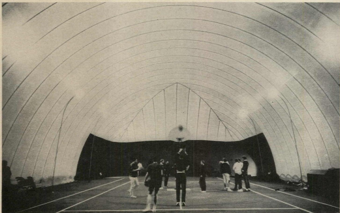
The pool bubble is 108 ft long, 68 ft wide and 31 ft high. A concrete ledge for anchoring the bubble runs along three sides of the deck and atop a concrete canopy extending from the building's side ( above ). Green plastic at the end walls of the athletic tent ( below ) provides contrast so that tennis players can see the small white ball
