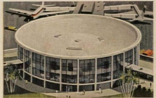
Resilient Barrett urethane insulation follows the contours of the "dish" roof on the Carson's O'Hare Airport restaurant in Chicago. Architect: C. F. Murphy Associates.
