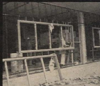
Then Keymesh Paperbacked lath is applied.
