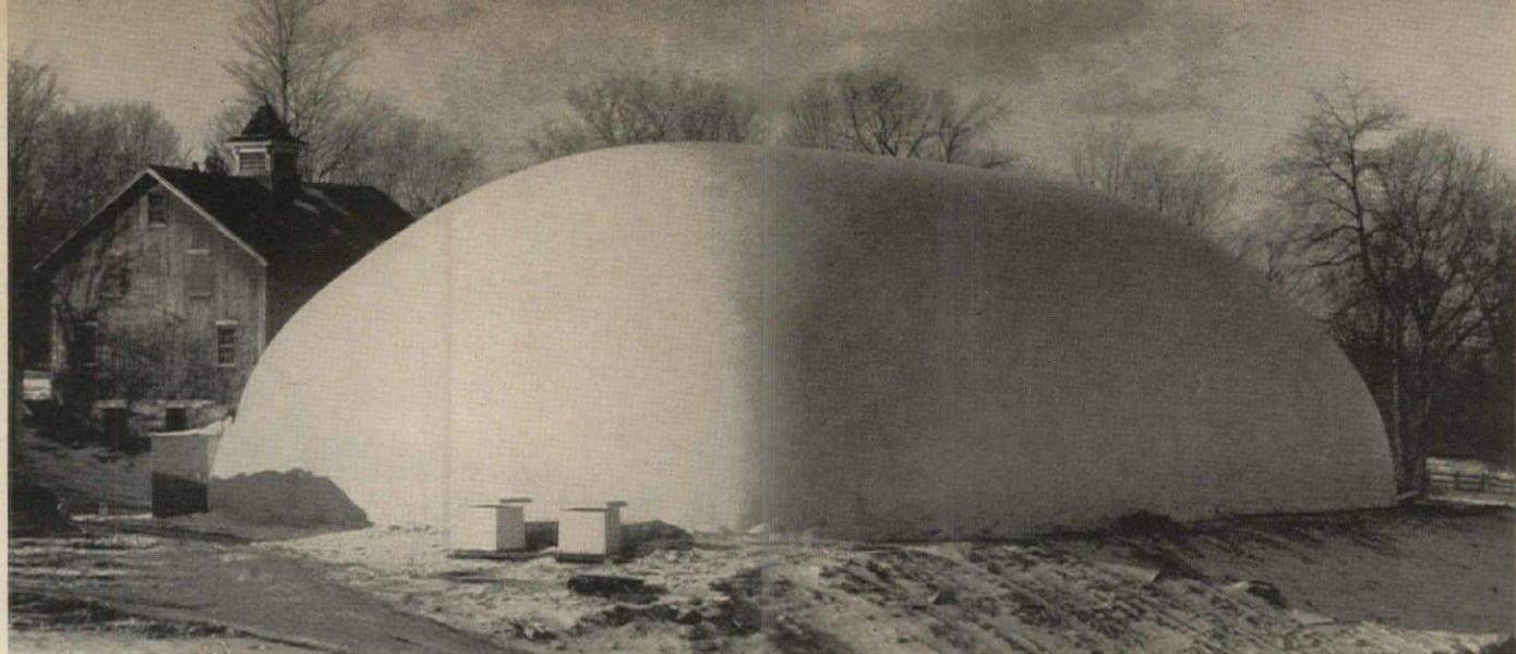
Two fans inflate and hold erect Forman School's unique gym in Litchfield, Conn.
