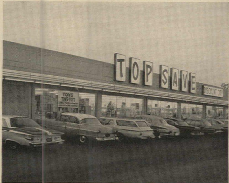
Top Save Store, located in Westgate Shopping Center, Streator, Illinois. 6 York SUNLINE units provide year-round comfort conditioning for this modern retail store.
