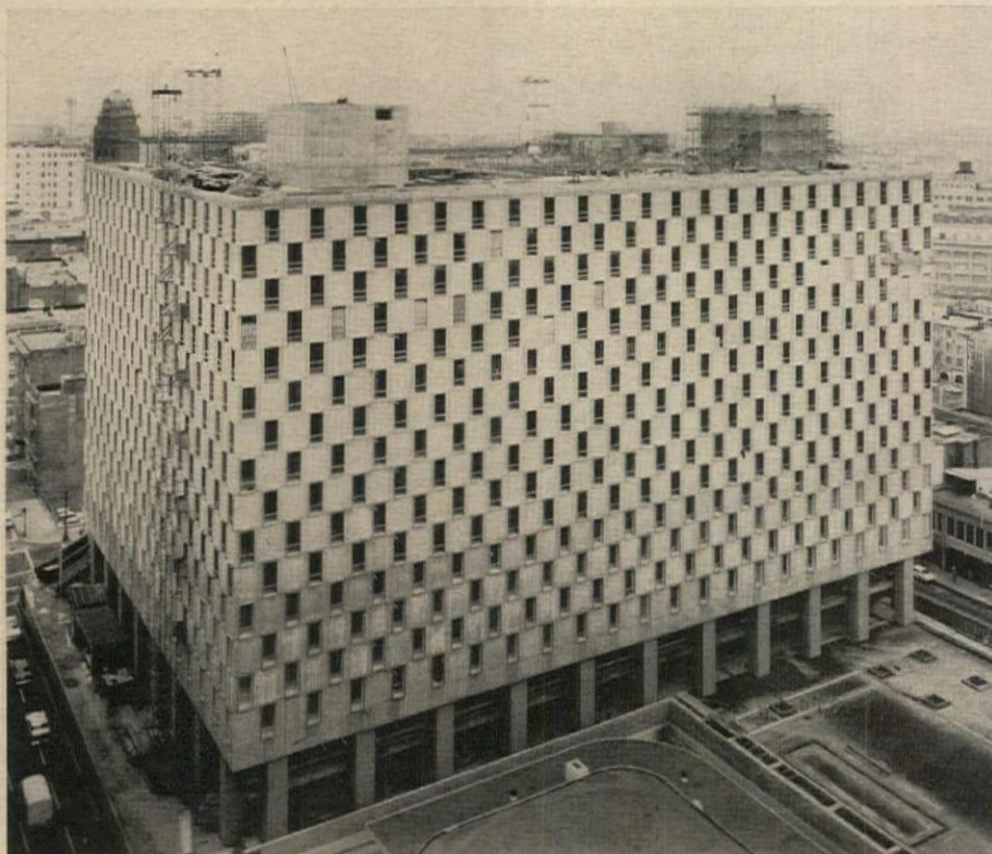
Hilton Hotel, San Francisco, California (left and above). Exposed exterior concrete frame walls are load bearing and serve as seismic-resisting elements. Even though the walls were increased 1 in. for every 25 ft of height after the first 15 ft, the wall analysis was based upon beam-column theories. The staggering of windows allowed straight-line placement of reinforcing bars along primary stress lines
