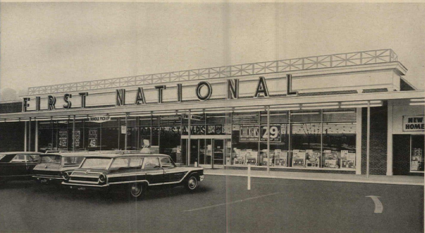
First National Store, Acton, Mass. Roof-mounted York SUNLINE units heat and cool entire store . . . take no floor space.
