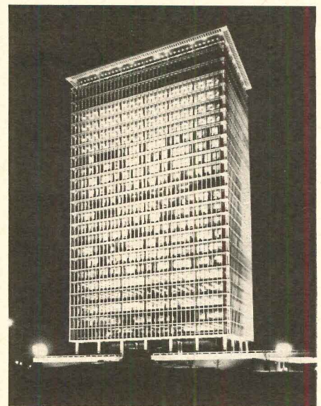
American General Life Insurance Building Houston, Texas Architects: Lloyd, Morgan & Jones Consulting Engineers: I. A. Naman & Associates Electrical Contractor: Howard P. Foley Company
