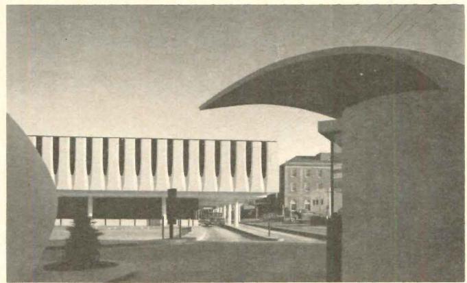
Six drive-in teller booths, connected by tunnel to the main building, are set under precast leaf forms echoing the dome
