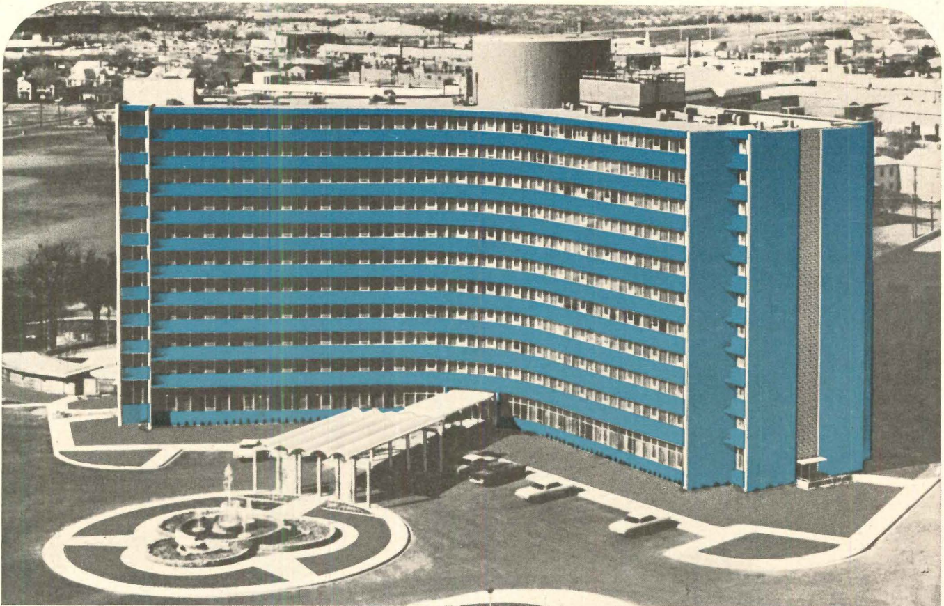
Photo courtesy of Reality Associates Ltd. Walter W. Ahlschlager, Dallas, Tex., architect
