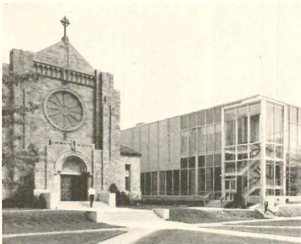
Some think that new buildings need not relate directly to the old
