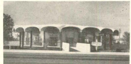
SECURITY FIRST NATIONAL BANK , Los Angeles, California. Architects and engineers: Welton Becket & Associates; structural engineers: Stacy & Skinner; general contractors: Del E. Webb Construction Company
