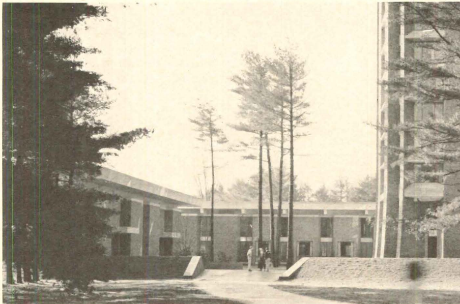
Main entrance to the Senior Center.
