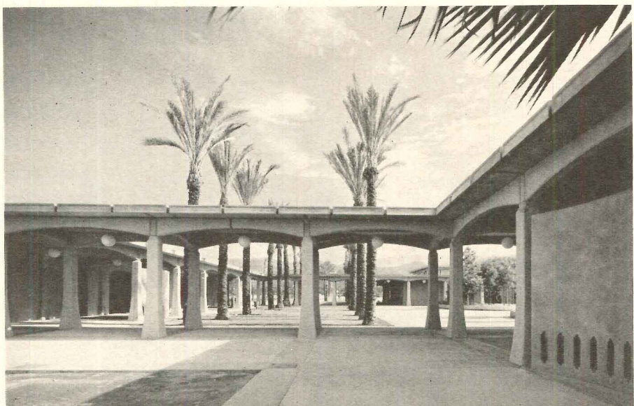
Shaped and sand-blasted concrete colonnades connect all elements of the campus
