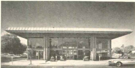
REDWOOD NATIONAL BANK , Napa Branch, Napa, California. Architects: Neill Smith & Associates; structural engineers: Gilbert, Forsberg, Diekmann & Schmidt; mechanical and electrical engineers: O'Kelley & Schoenlank; general contractors: D. M. Christensen Construction Company
