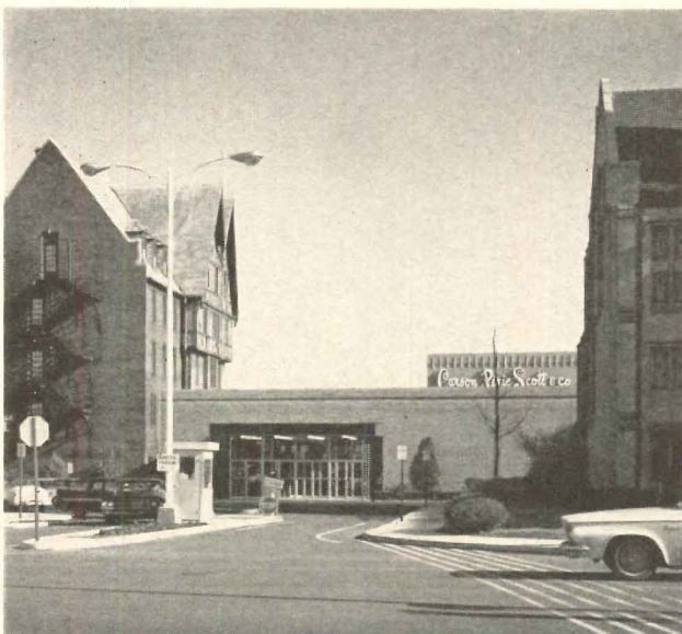
Combination of old and new: one of the arcade entrances
