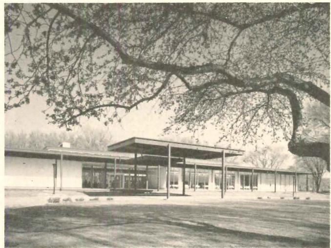
Club house at Old Orchard Country Club, a daily-fee golf course in Prospect Heights, Illinois, is designed around a simple steel structural system. Nearly all-glass walls are set back 10 feet from the roof line to form a shaded arcade all around the building. Architects: Alper and Alper; structural engineers: William S. Silberberg & Associates.
