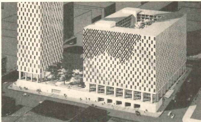
Rendering shows cross-bracing reinforcement
