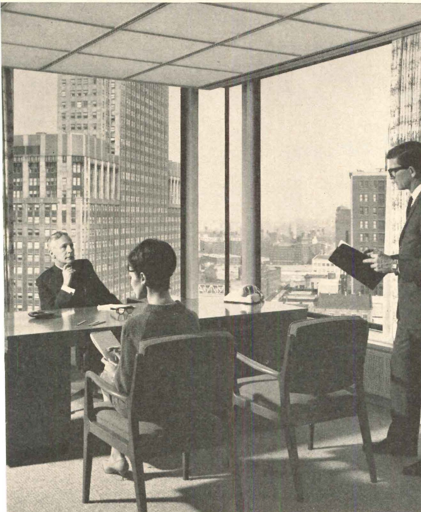
Heavy-Duty Parallel-O-Grey® Plate Glass was selected for its glare- and heat-reducing properties, and is ⅜"-thick for strength requirements of the design.
