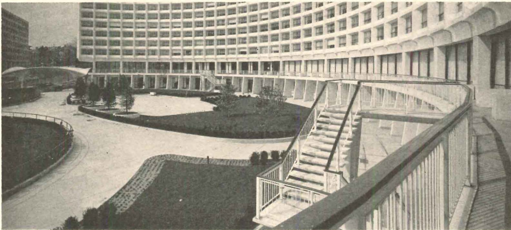
Resort plaza over parking is faced by two tiers of lanai rooms
