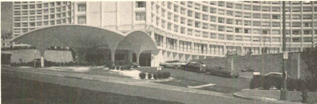
Canopied ballroom entrance to lower lobby with ramp to parking
