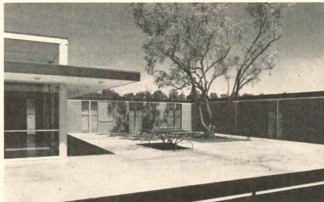
Walls around open spaces have grill inserts for ventilation
