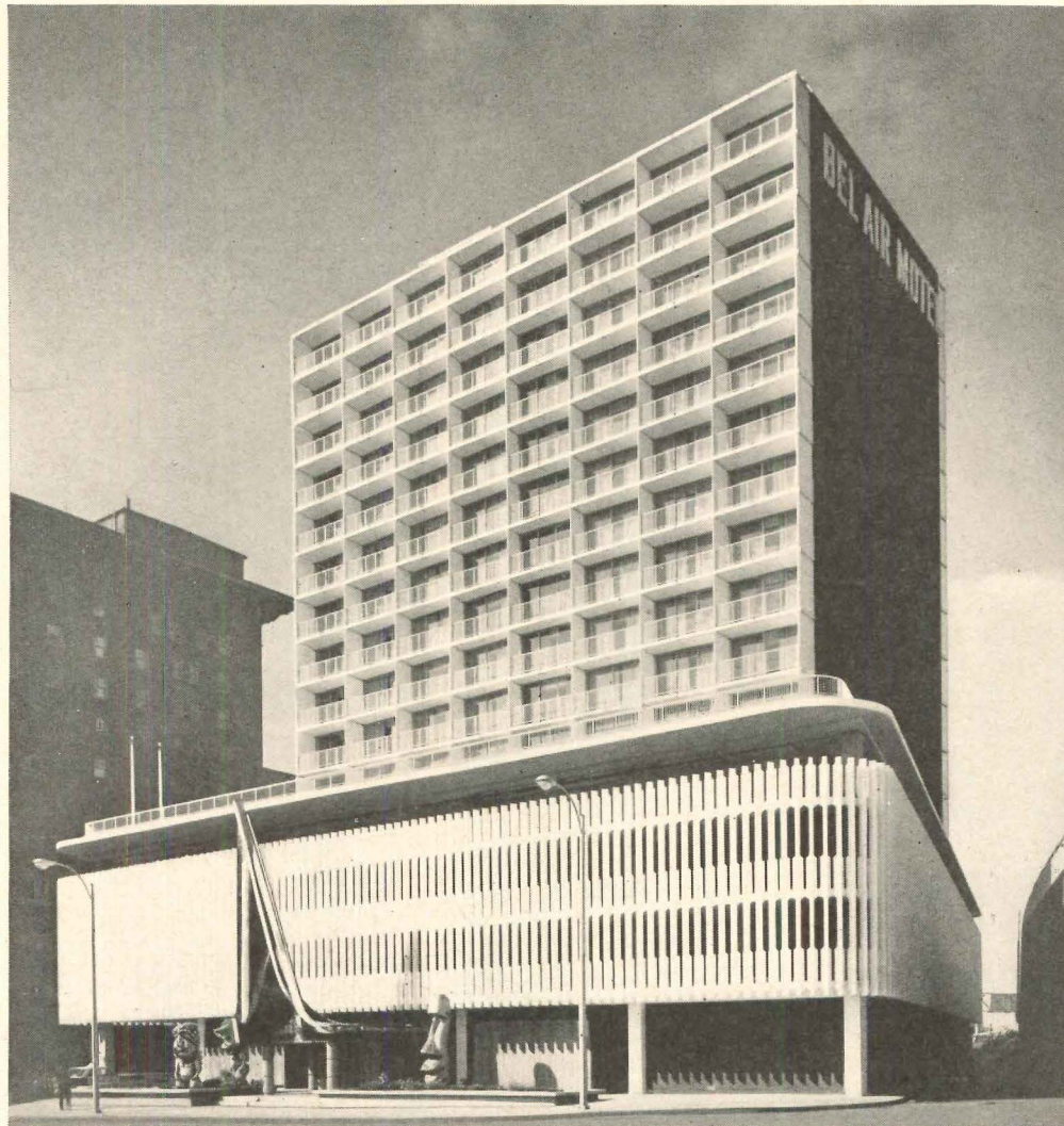
BEL AIR EAST MOTOR HOTEL , St. Louis, Missouri, is completely air conditioned by a York central system with individual room control for guests. Owner, Boulevard Investment Company; Architect, Hausner & Macsai, Chicago; General Contractor, Westlake Construction Company; Consulting Engineer, William Goodman, Chicago; Mechanical Contractor, Natkin & Company.
