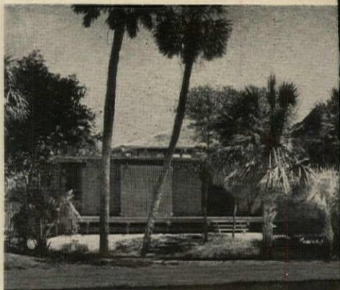
Architects: McGinty & Stanley
