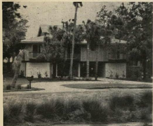
Architects: McGinty & Stanley
