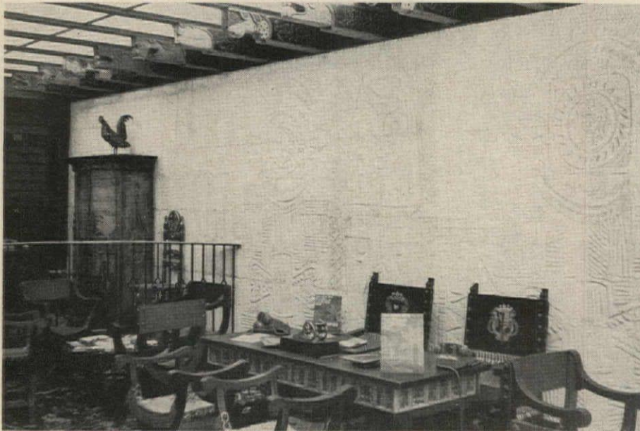
The use of a luminous ceiling in this space produces a diffuse non-directional source of light, so that the elaborately sculptured wall is washed almost flat because of the lack of shadows. Angled, directional lighting focused on the wall would have brought the sculptured designs into sharp relief.
