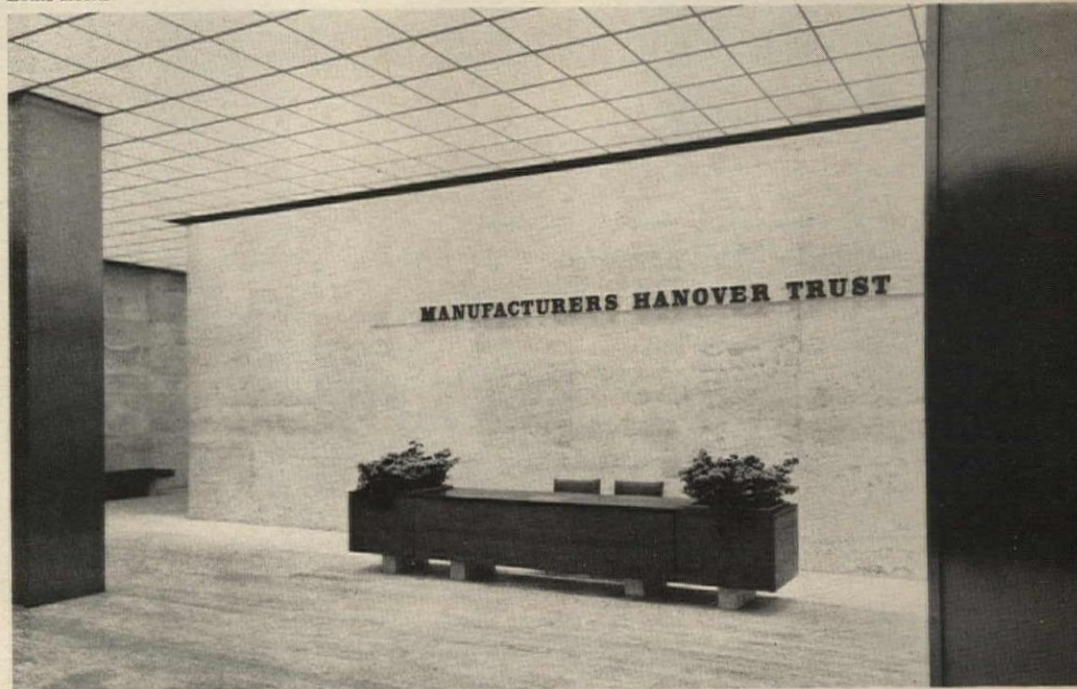
Wall wash lighting of the focal wall of this lobby achieves good distribution from top to bottom without hot spots or shadows from the fixture. The matte surface of the travertine eliminates light source and other confusing reflections.
