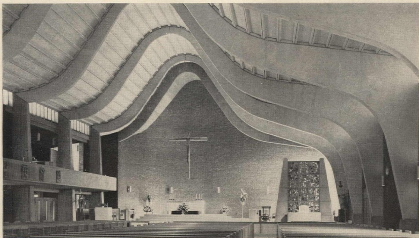
The curving roof is high to accommodate the choir loft over the "Crying Gallery," reaches its peak on the axis perpendicular to the main altar and quickly descends to provide an intimate low roof over the section reserved for private prayer and contemplation of the Blessed Sacrament. A careful attempt was made to emphasize in plan and function the primacy of the Mass.
