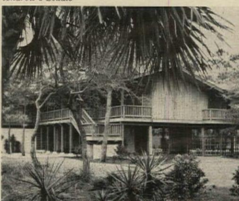
Architects: McGinty & Stanley
