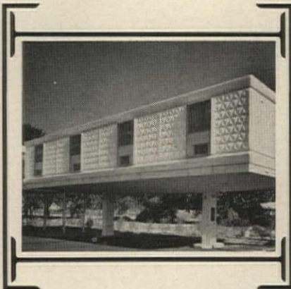
Holiday Inn Jr. Motel, Memphis, Tennessee, has a J&L lightweight structural framework to resist deflection both for cantilever loading when in place and for over-the-road hauling.
