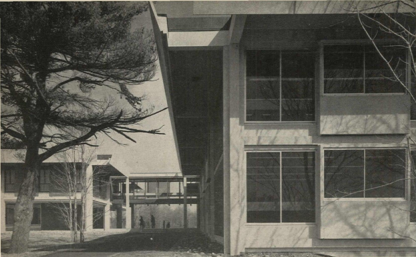
CORNING COMMUNITY COLLEGE, Corning, New York; Architects: WARNER, BURNS, TOAN, LUNDE, New York; Structural Engineers: SEVERUD-PERRONE-FISCHER-STURM-CONLIN-BANDEL, New York; General Contractor: ROGER & McCAY, INC., New York; Precast, Prestressed Concrete: FORMIGLI SALES COMPANY, Philadelphia, Pa.
