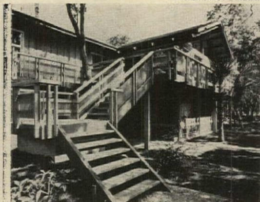
Architects: McGinty & Stanley
