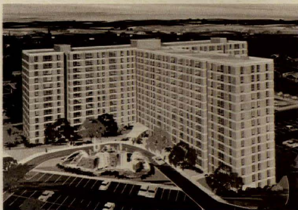
Use of rigid urethane foam as structural insulant for $8-million apartment complex reduced construction costs, could shave $2000 a year from heating and cooling bills.
