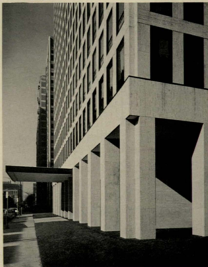
Detailing of the building shows the simplicity and precision that mark most SOM designs. The building is clad with Roman travertine, windows are grey glass. Lower floors have complete shopping facilities.
