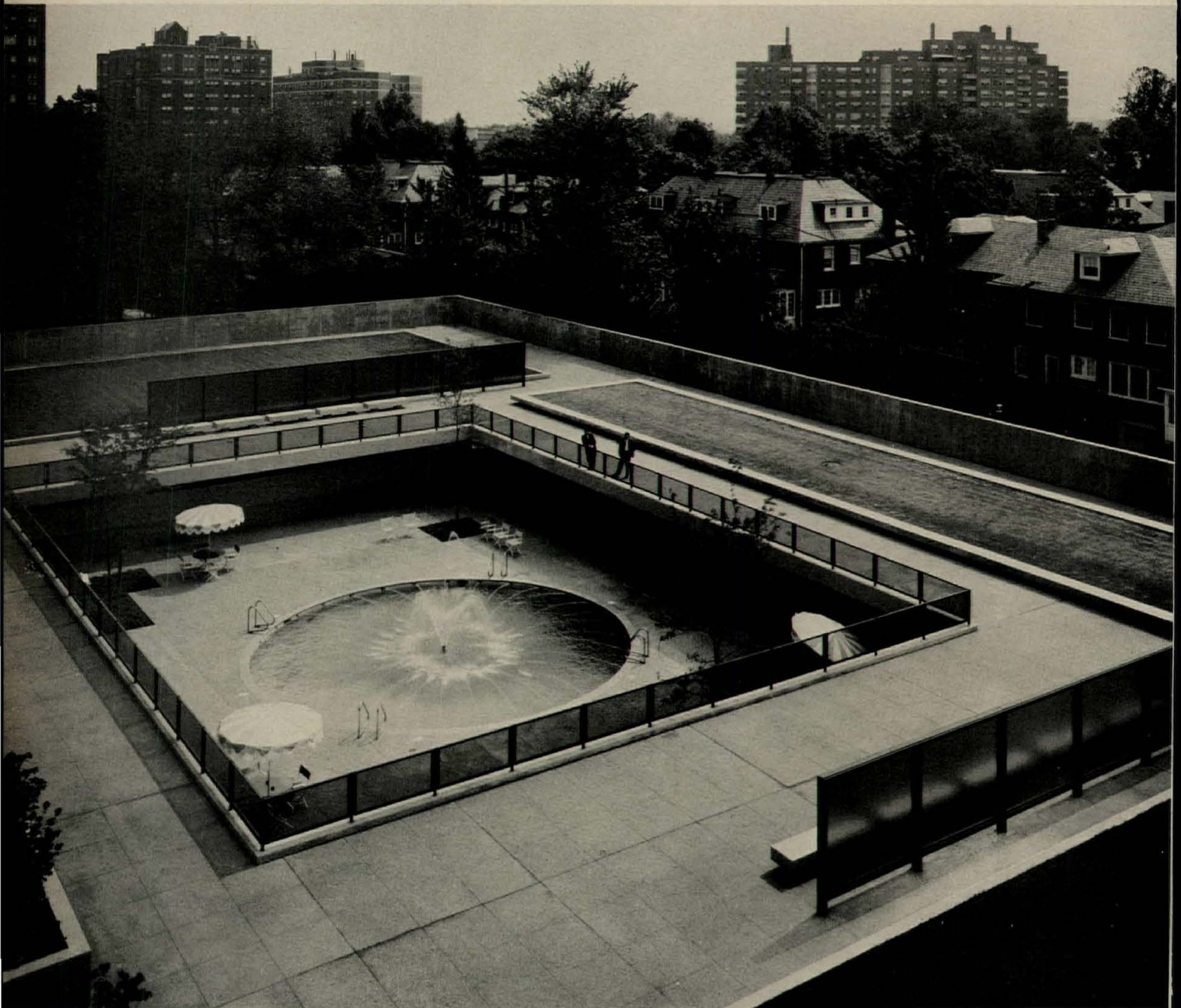
The above-grade plaza is isolated from the neighborhood by high walls. Walls of planting beds and free-standing benches provide plenty of seating area. Paving is a warm buff color.
