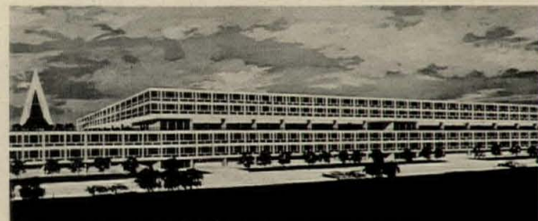
Three- and six-story quarters will be built in two increments of 307,500 square feet and 324,778 square feet, to provide a total of 832 two-man rooms.
