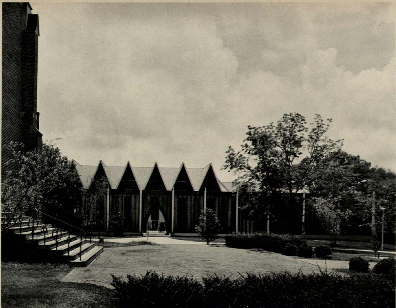
DANA FINE ARTS CENTER at Agnes Scott College conceals complicated interior spaces behind decorous neo-gothic screens. Frankly ornamental, the screens echo architecture of older college buildings. (October 1965, pages 158-160.)
