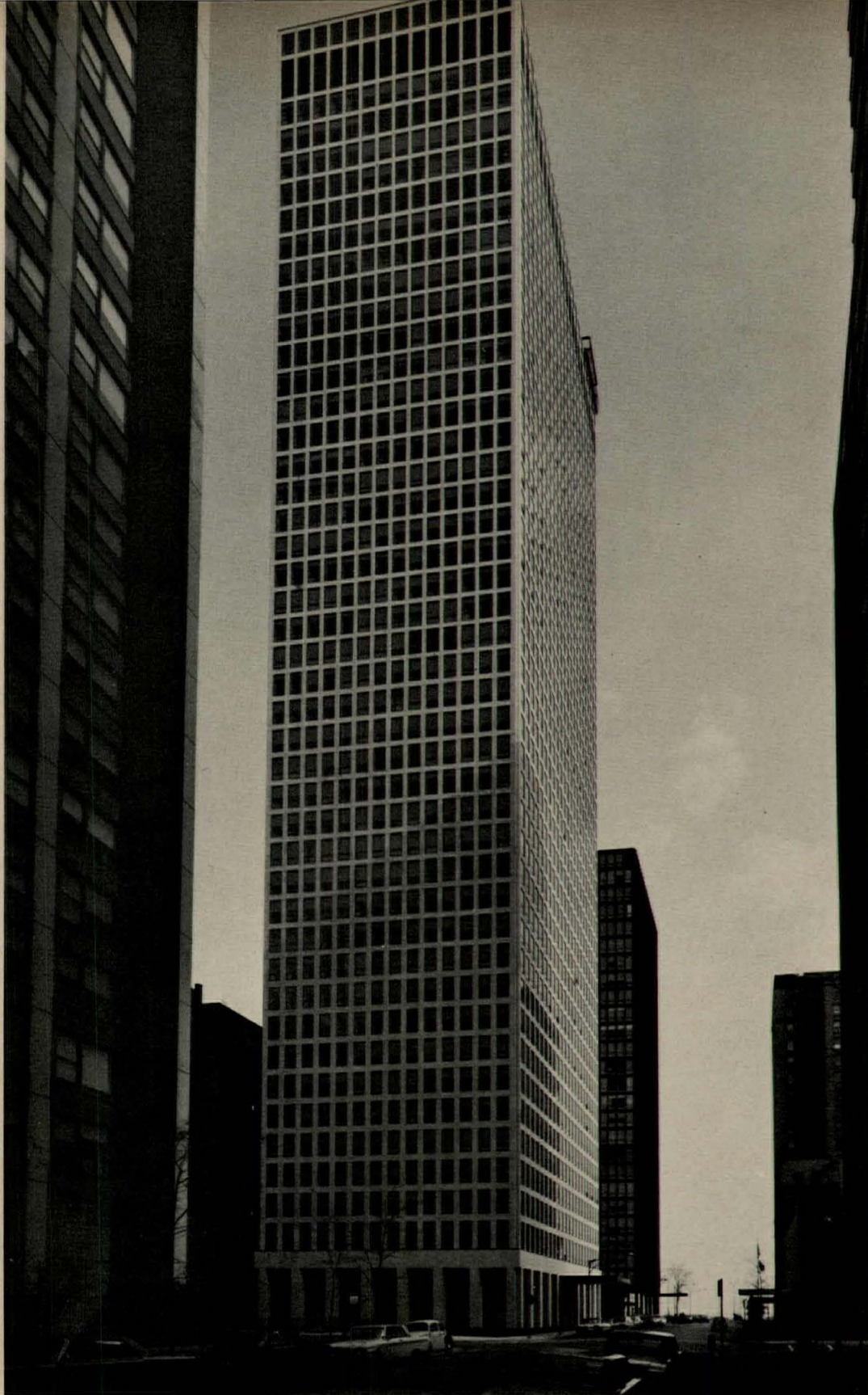
Closely spaced exterior columns eliminated shear walls, permitted great planning flexibility.
