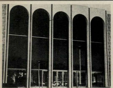
Custom factory fabrication was required for the 1/2-in.-thick, pattern-cut tinted lights for this department store.
