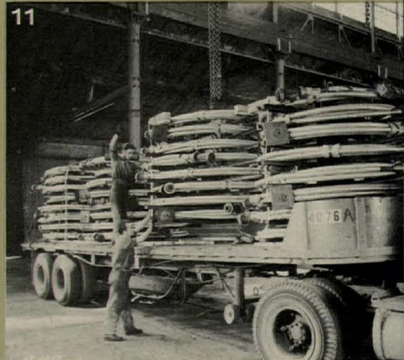
11. Rotatable shipping racks give protection to coiled tendons enroute, minimize storage space requirements at job site and simplify handling and placement.
