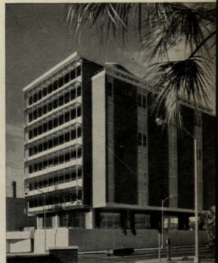
TAMPA, FLORIDA: 8-story, 97,000 sq. ft. IBM office building. Architect: Aeck Associates. Engineer: Blakely-Daniels and Associates. Contractor: International Construction Co.
