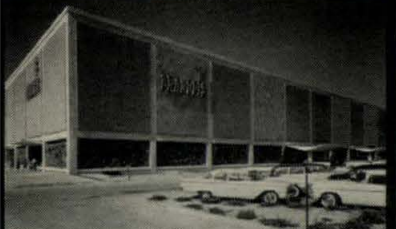
Brandeis Department Store — Omaha Architect: Leo A. Daly-Omaha. Terrazzo Contractors: Demarco Brothers Co. and Universal Terrazzo & Tile Co. Jointly-Omaha.
