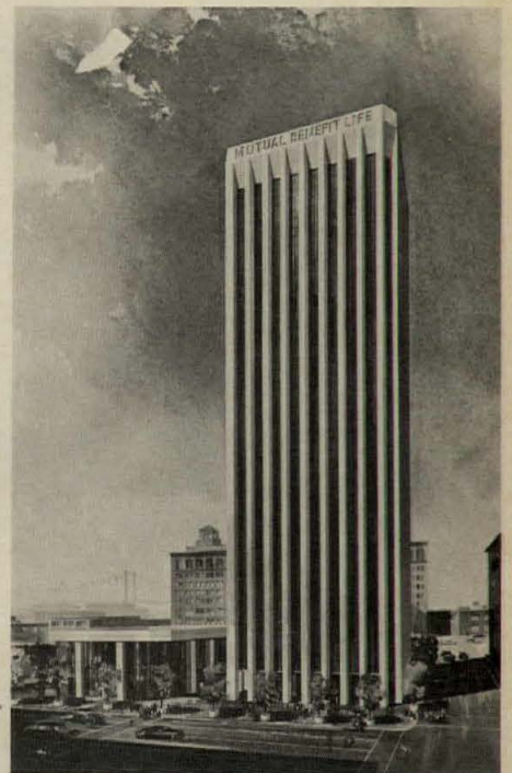
An office building in San Francisco for the Mutual Benefit Life Insurance Company, designed by Welton Becket Associates, is supported by 4-foot-10-inch-wide white prestressed concrete columns framing bronze-anodized aluminum windows twice as wide as the columns. The 32-story office tower will contain 575,000 square feet of office space with parking in the basement, and a two-story annex will contain 15,000 square feet of office space. The entire weight of the structure will be borne by the outside columns and the central elevator shaft, providing column-free interior space. General contractor will be Haas & Haynie Corporation.
