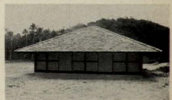
Simple detail and careful design produced houses for $14,000 each, half usual government house cost.
