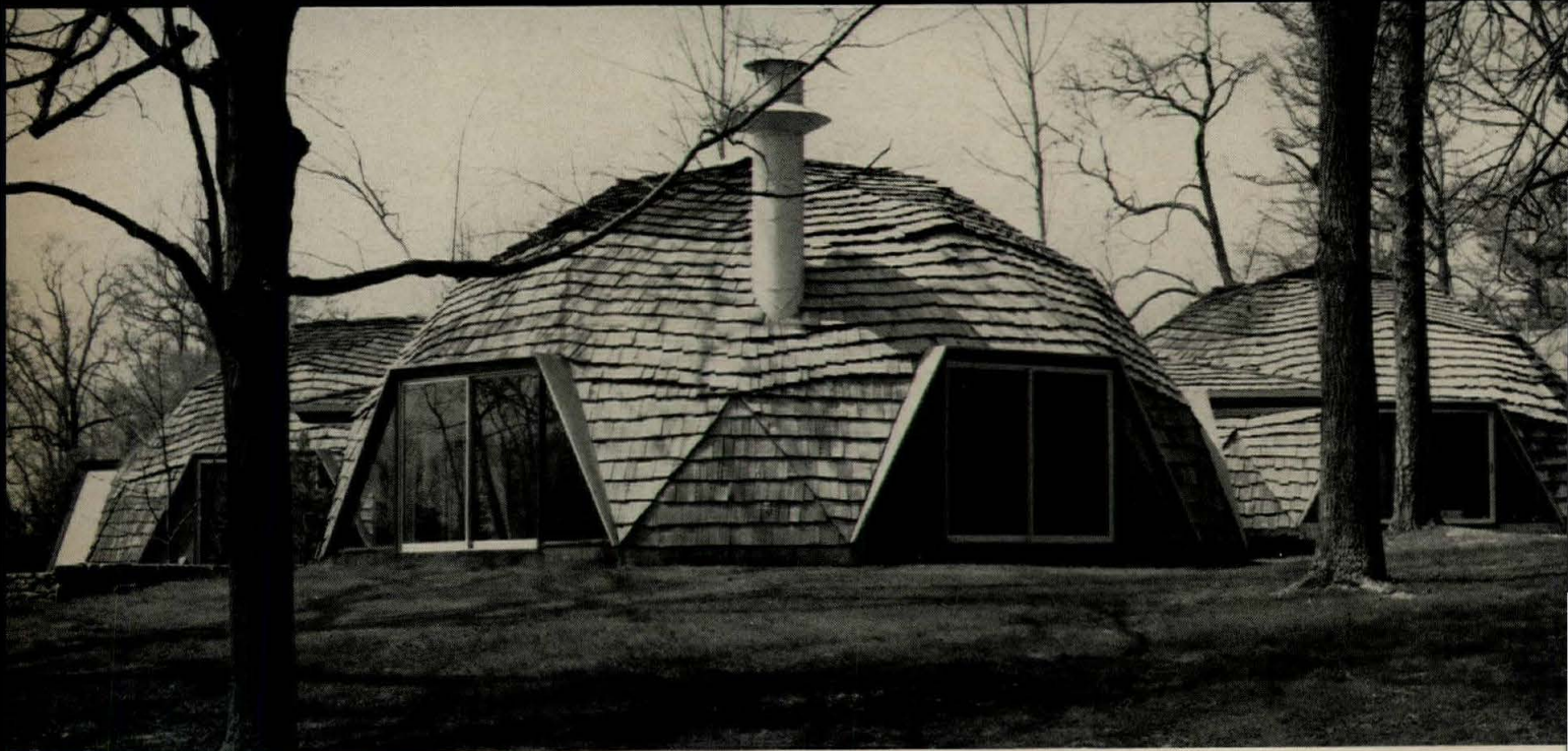
Residence, Narberth, Pennsylvania Architect: Stein and Rowland Associates Certi-Split Handsplit-Resawn Shakes, 24" x 1/2" to 3/4" with 8" to 10" to the weather.
