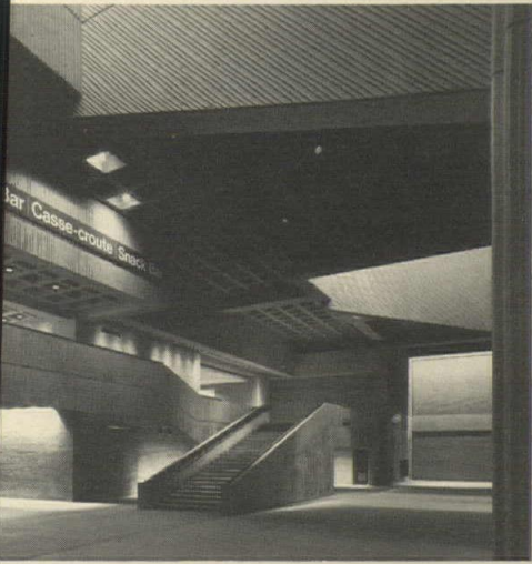
Place Bonaventure , a massive trade center downtown Montreal, should be seen by architects during the trip to Expo. Shown below is its vast exhibition space. Giant columns support eight floors above.
