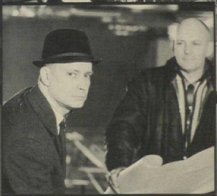
Architect Charles H. Harper (left) discusses floor installation with James Lawton, job foreman for general contractor, Joseph P. Jansen.
