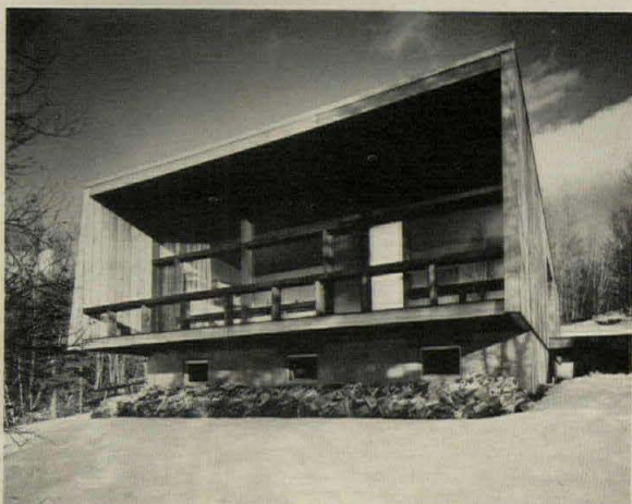
Deeply set-back porch with cantilevered deck provides additional summer living space, cross-ventilation and an impressive view to the west.
