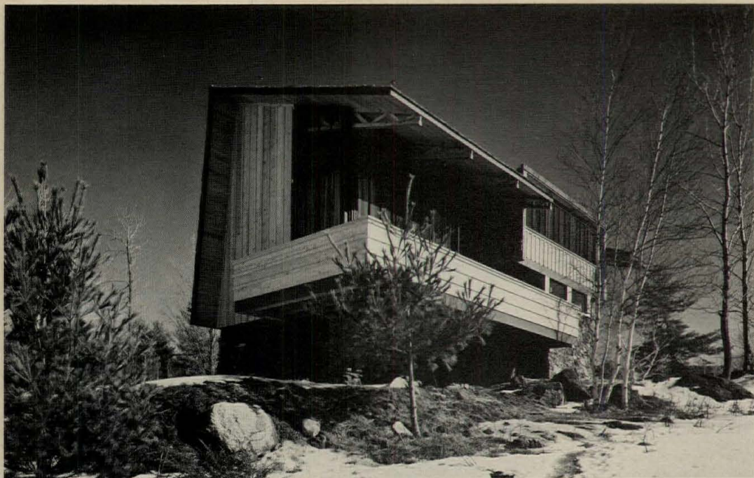
The ski lodge is oriented to a southerly view and the large porch extends a multi-purpose living area for summer use.
