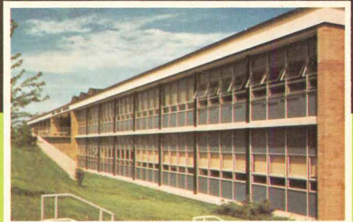
Fort Crook School, Omaha, Nebraska Architect—Martin, Money and Assoc. Contractor—Butler Construction Co.
