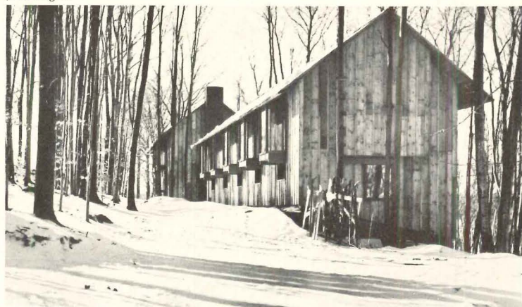
Girls Dormitory, Putney School , Putney, Vermont. Architect: John B. Rogers. "The non-institutional character and the strong sense of structure (partly student-executed) overcome any lack of skillful finish or small inconveniences. Outside, one of the particularly delightful features is integration of building with landscape and an awareness of line: their fine, upstanding exterior effect, their harmony with the thin lines of trees, and the thin winter shadows cast by the trees in wintry country." Structural engineers: Souza and True.
