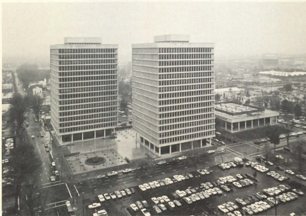
The new high-rise office buildings in the foreground are just two of the 15 buildings served by a huge $13-million central heating and cooling plant (low building at right) and distribution complex. The central plant supplies steam
