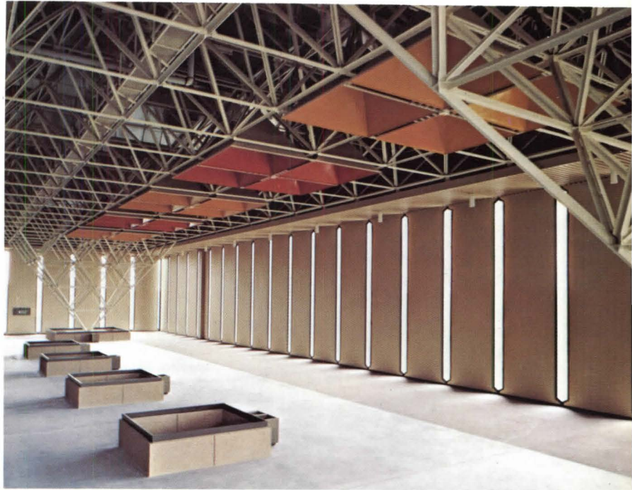
The Bethlehem Mayari R panels are constructed with painted sheet steel panels on the inside.
