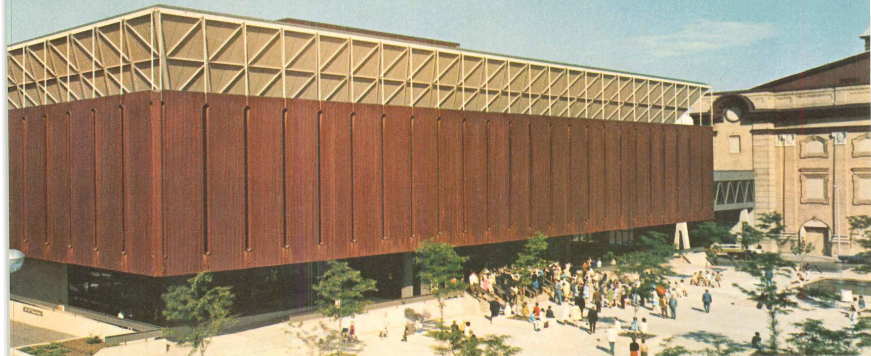
Currihan Exhibition Hall, Denver —"This building is distinguished by its tremendous space frame that gives the entire structure a sense of dramatic power. The interior expression is particularly impressive."
