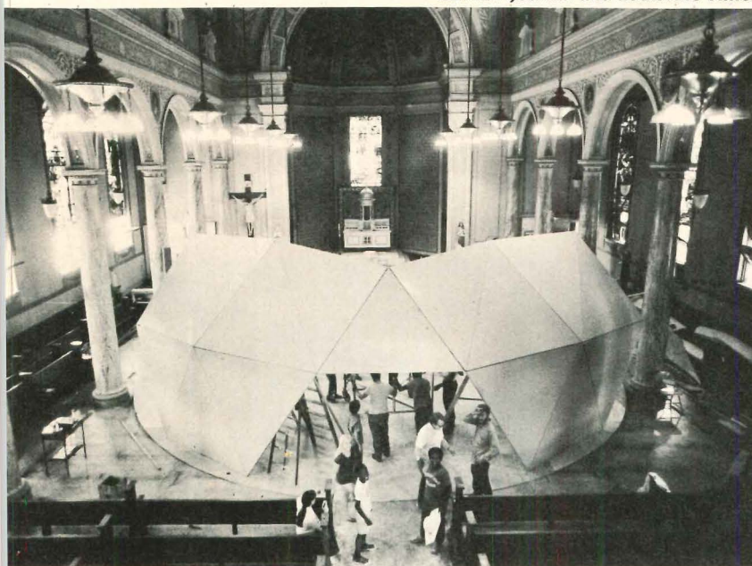
St. Charles Borromeo Catholic Church renovation, Louisville, Ky., Jasper Ward, architect, was designed to meet the needs of a reduced congregation in a large ghetto church. A geodesic dome,
