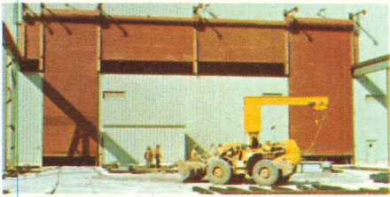
MOTOR OPERATORS OPEN THE DOORS BY ACTUATING SEQUENCE TYPE ELECTRIC CONTROLS.
