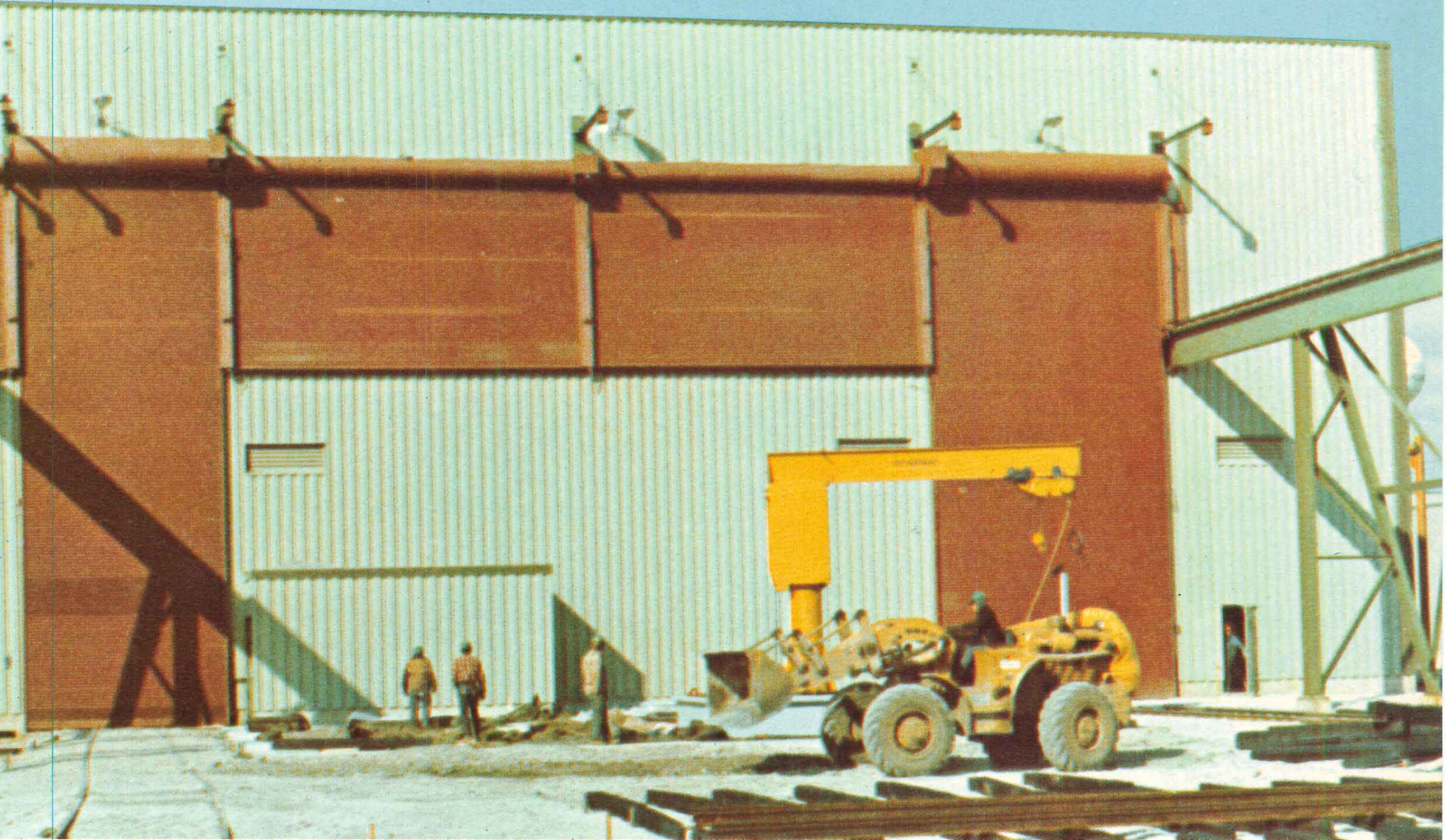
THIS LARGE CRANE OPENING IS COMPLETELY CLOSED WITH KINNEAR MOTOR OPERATED DOORS.
