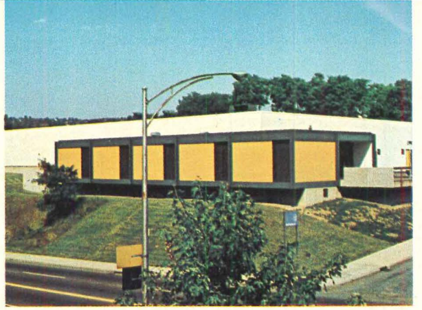
Westinghouse Electric Corporation Homewood Plant, Pittsburgh, Pa. Architect: Walter Roberts Associates, Pittsburgh, Pa. C-Panel System, 4" and 8" Ribbed Exterior Profile.
