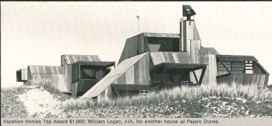
Residential/Single-Family Buildings Top Award $1,000: William Logan, AIA, (Neil Noll, Mike Lee Associates, Palo Alto, Calif.). Project: House at Pajaro Dunes, Watsonville, Calif.
