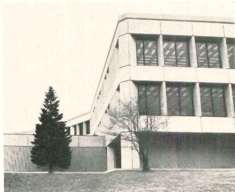
Detail of interesting exterior with exposed reinforced concrete sandblasted for texture.
