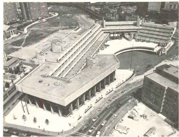
Aerial perspective photo of the State Service Center, tower unbuilt
