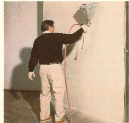
attractive, textured finish coat is sprayed over the prime coat. Both prime and finish coats can be troweled or sprayed. The result is superior insulation and the attractive finish shown at the right.
