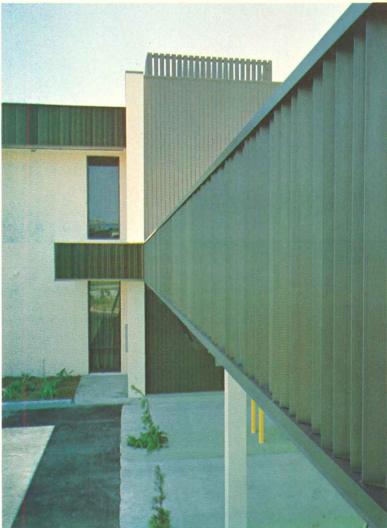
Project: Guardian Bank, Pinellas Park, Florida Architect: Robert Bernzott Fabricator: J-C Products Corporation Applicator: Midway Glass Company
