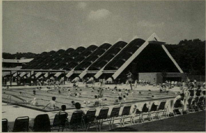
ECHO PARK POOL COMPLEX, Long Island, New York
