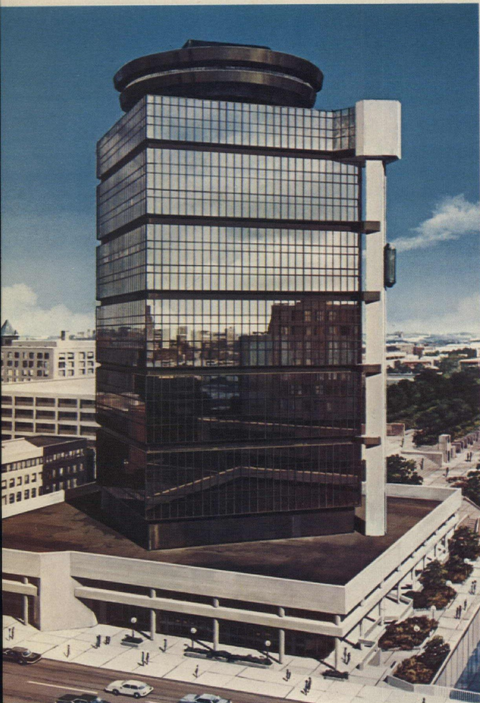
Architect's rendering depicts the First Federal Savings and Loan office building in Rochester, N.Y. When completed in late 1976, the structure will feature a revolving roof-top restaurant, an outside glass-enclosed elevator, and a mirror exterior which will reflect the surrounding community.
