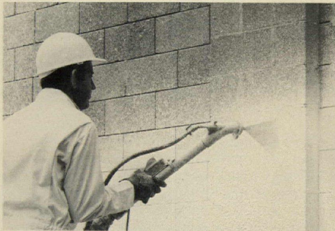
Spraying is the fastest way to apply BlocBond. Three men can cover about 1200 sq. ft. an hour.
