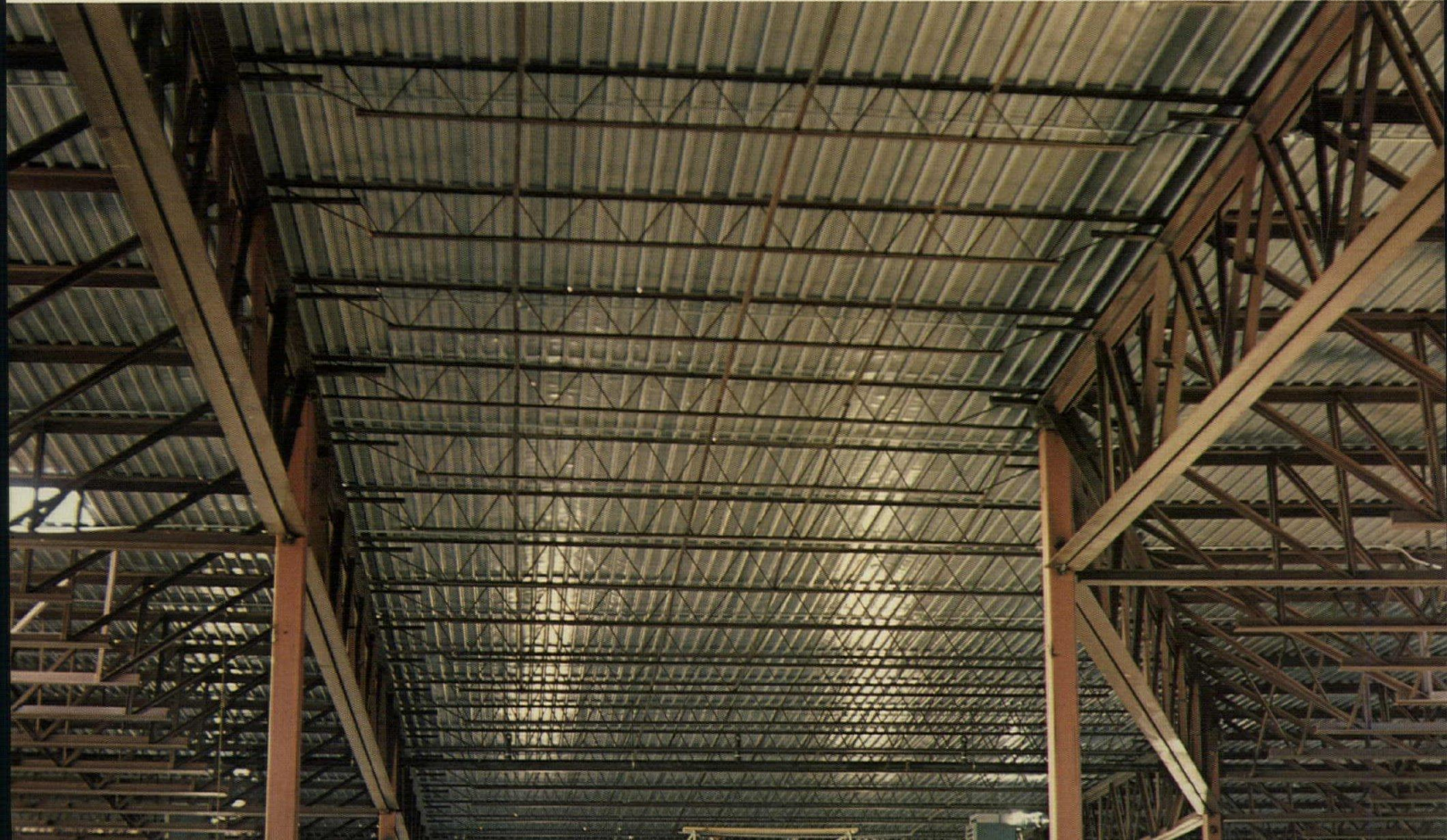
Joist girders were engineered and designed to meet the particular requirements of this job.
