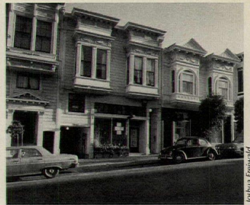
Sacramento Street Apartments, San Francisco. Kaplan/McLaughlin, Architects, Planners
