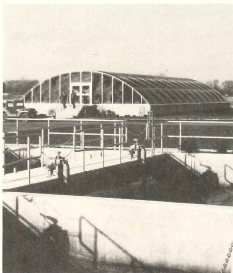
WATER TREATMENT PLANT, Crystal Lake, Illinois
