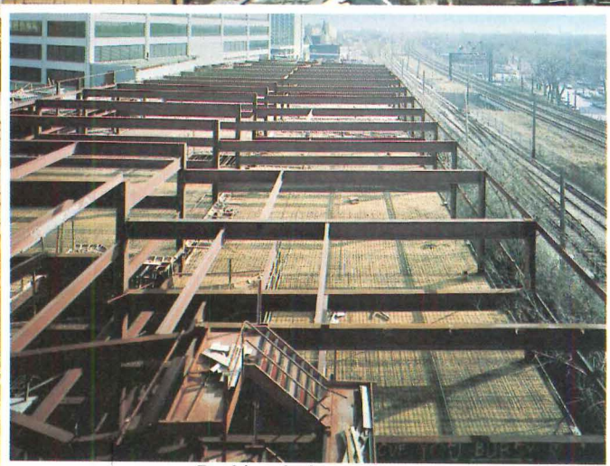
Parking deck structure.
