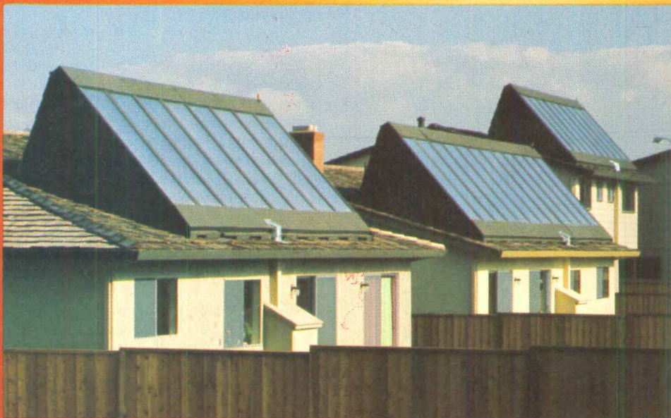
Solar heating development at Laurel Park East, Santa Clara, California, utilizing tempered Sunadex™ glass Collector manufactured by American Solar King, Inc.
