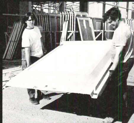
Construction workmen demonstrate light weight, ease of handling of 7' x 5' aggregate faced building panels of GRC.
