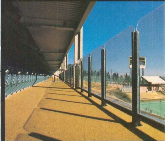
Spectator glazing protects without obstructing view of game at University of Colorado Stadium, Boulder, Colorado. Architect: Herb Ross.
