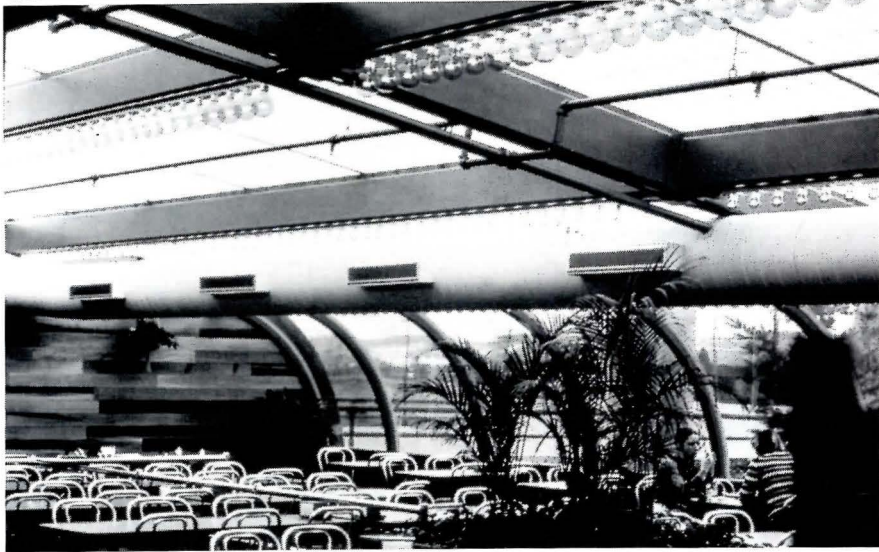
The translucent "skyroof" over this fast-food restaurant in Portland, Oregon is the first application of a translucent roof covering that has a Class "A" U.L. listing (for severe fire exposures). It comprises fiberglass-reinforced plastic skins bonded to an aluminum grid by Kalwall Corporation. Architects: Boutwell, Gordon, Beard & Grimes.
