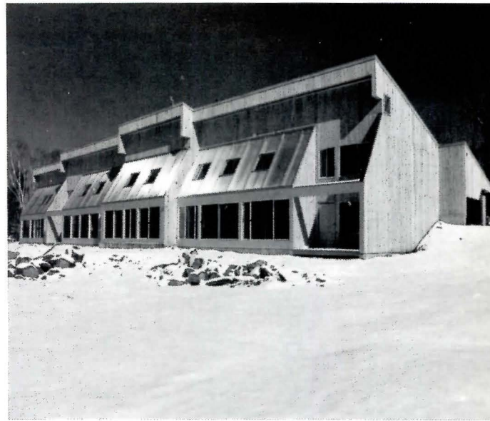
Sloped glazing for passive solar in this housing at White Mountain School in New Hampshire has clear panels for a view of the sky in the midst of a large area of panels comprising acrylic double-skinned sheet made by Cy/Ro Industries (winter U value is 0.58). Architects: Banwell, White and Arnold.
