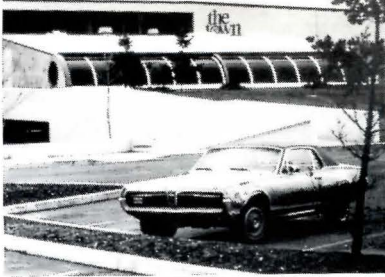
The translucent "skyroof" over this fast-food restaurant in Portland, Oregon is the first application of a translucent roof covering that has a Class "A" U.L. listing (for severe fire exposures). It comprises fiberglass-reinforced plastic skins bonded to an aluminum grid by Kalwall Corporation. Architects: Boutwell, Gordon, Beard & Grimes.
