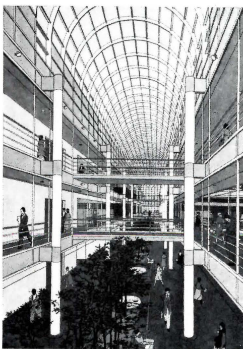
A long gallery gives relief to large open-plan areas and provides an interior street in AT&T's 400,000-sq-ft Long Lines Eastern Area Headquarters, Oakton, Virginia, designed by Kohn Pedersen Fox Associates, Architects. To meet energy-code requirements, reflective insulating glass was used throughout, and a large portion of the curvilinear cafeteria enclosure has opaque insulated panels. Insulating glass is heat-strengthened, and the inboard light is laminated. Skylight fabricator: Super Sky Products.
